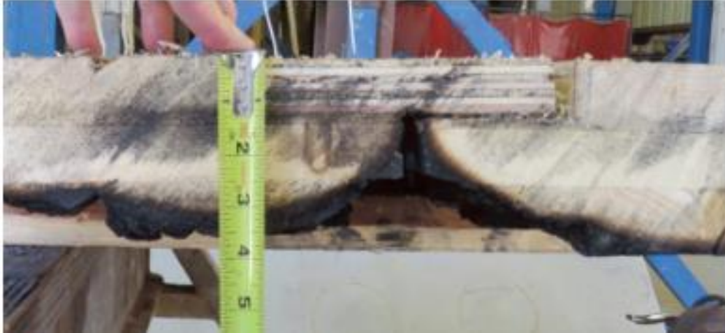
Figure 2.2. CLT Degradation Near Fastener (Barber et al., 2022)
