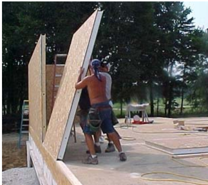
Figure 4-3 SIPs construction needs few braces. Photo courtesy of Fischer SIPs.
