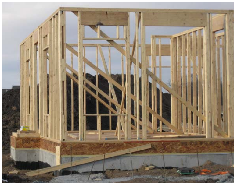
Figure 2-1 Walls in place of a stick framed structure
