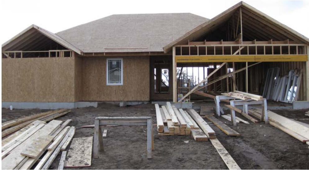
Figure 6-5 Construction site of a new stick built house
