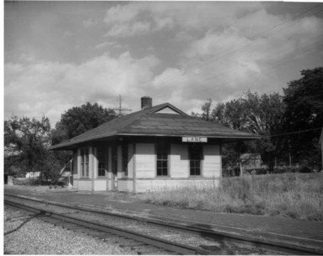
Figure 3. A historic photograph of the Lane, Kansas train depot on the Missouri Pacific Railroad. C. 1918. This is possibly the original Avondale station, with the addition of a sign that says "Lane". SOURCE: Repository: kansasmemory.org
