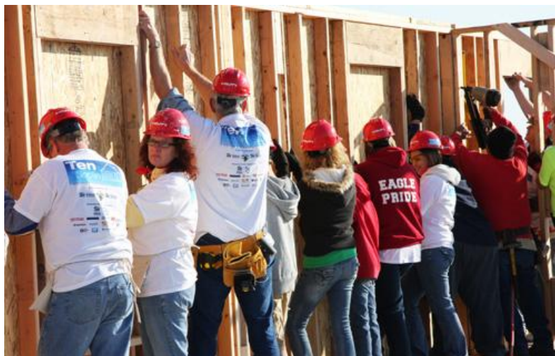
Figure 8: Ten For Joplin Raising Walls.
