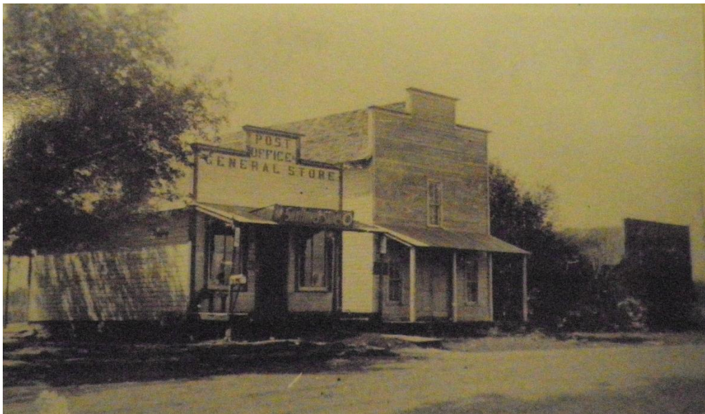
Figure 2. The general store and post office.
