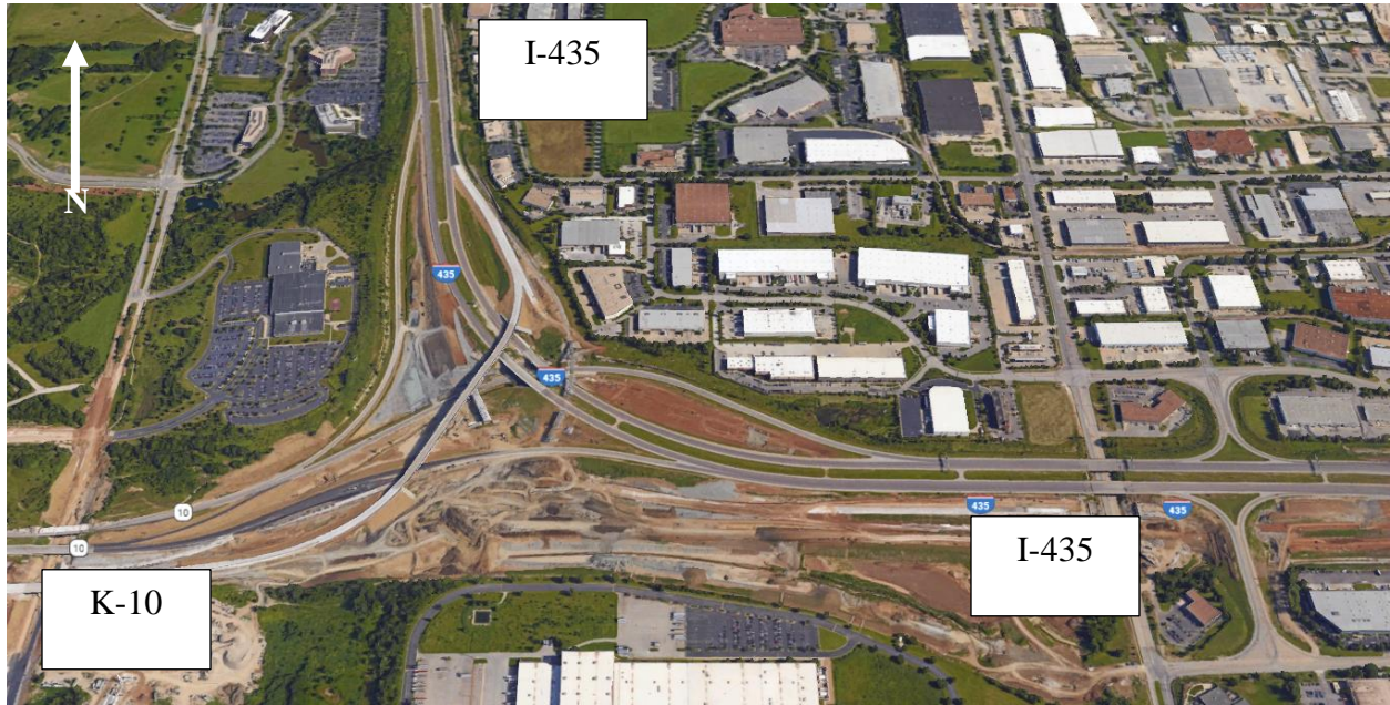
Figure 17 Google Maps Image of Gateway Project Construction (Google Maps, 2017)
