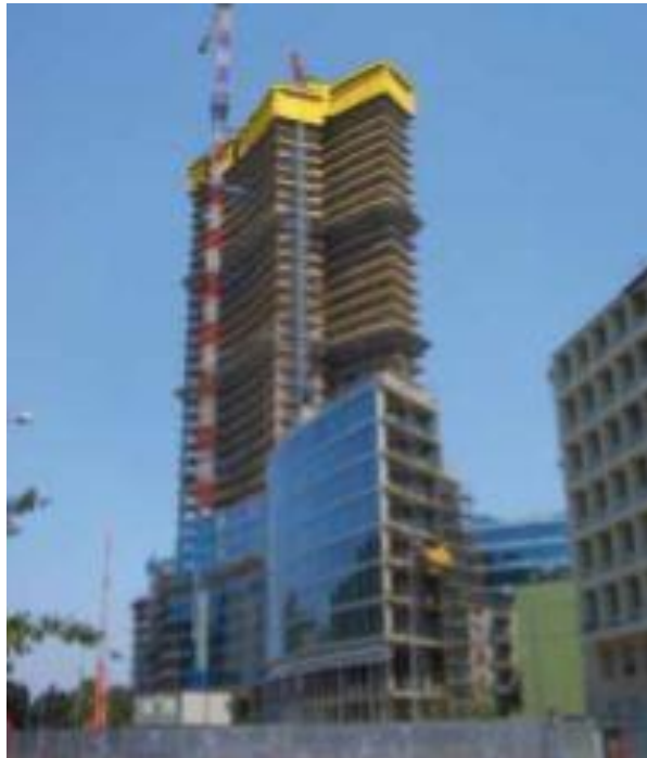
Figure 5-5: Palazzo Lombardia During Construction ( Cobix Insight, 2010 )
