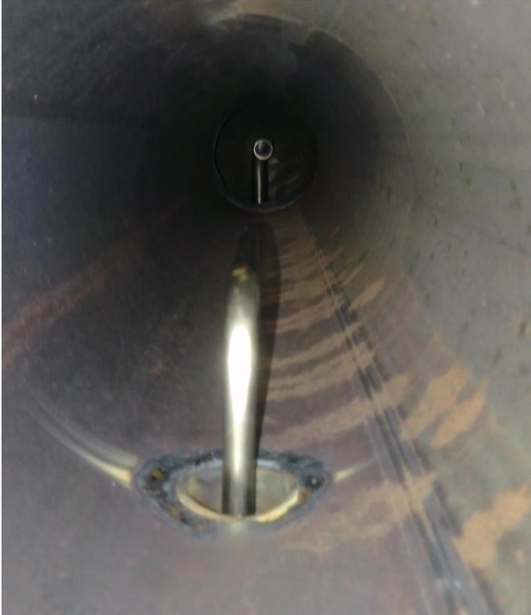
**Figure 3-3 C18 Oil Injection and Sample Ports**
