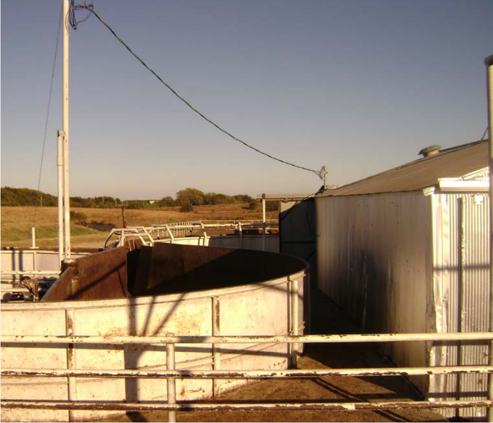
Figure 5.20 Knight Feed Yard, Light pole at south load/unload cause of triggers and interference noted it Figure 5.18.
