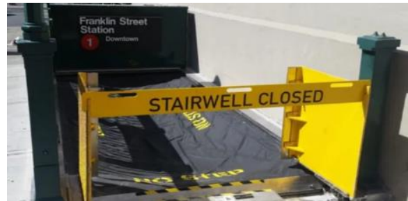
Figure 23: Flex Gate at Franklin Street Station
