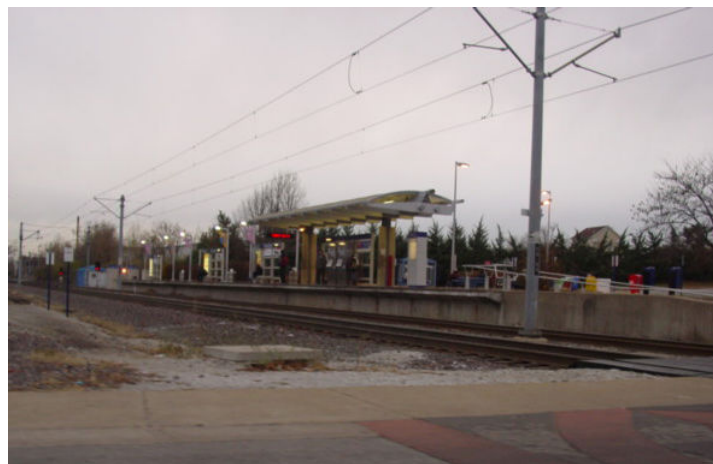
Figure 4- 5 Wellston Metrolink Station
