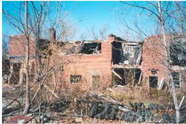
Figure 4- 16 Abandoned building on ABEX Foundry site
