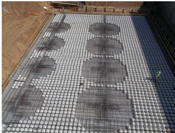
Figure 5-3: Bubbledeck Voided Slab at Labahn Hockey Arena
