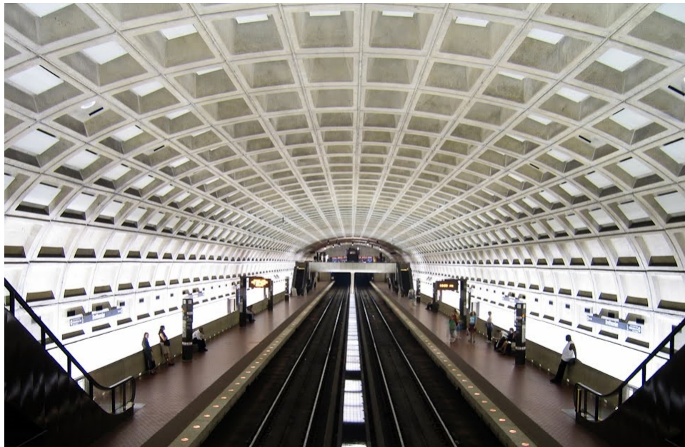
Figure 2-2: Waffle Slab in Washington DC Metro Station
