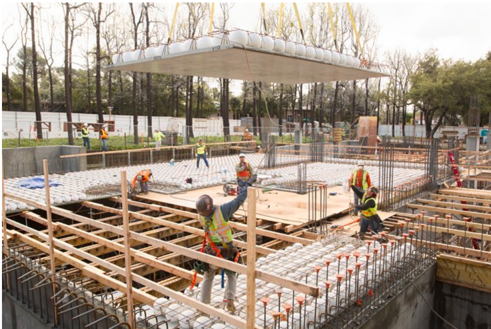
Figure 5-4: Semi Pre-Cast Voided Slab Construction at Harvey Mudd College
