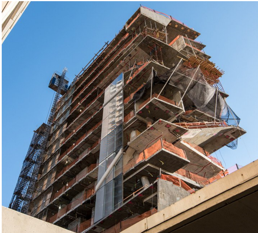
Figure 5-2: CUMCGEB Cantilevered Flat Plate Voids Slab
