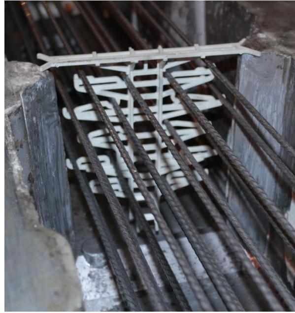
Figure 78 Wire “chair” supporting 5.32-mm. diameter wires
