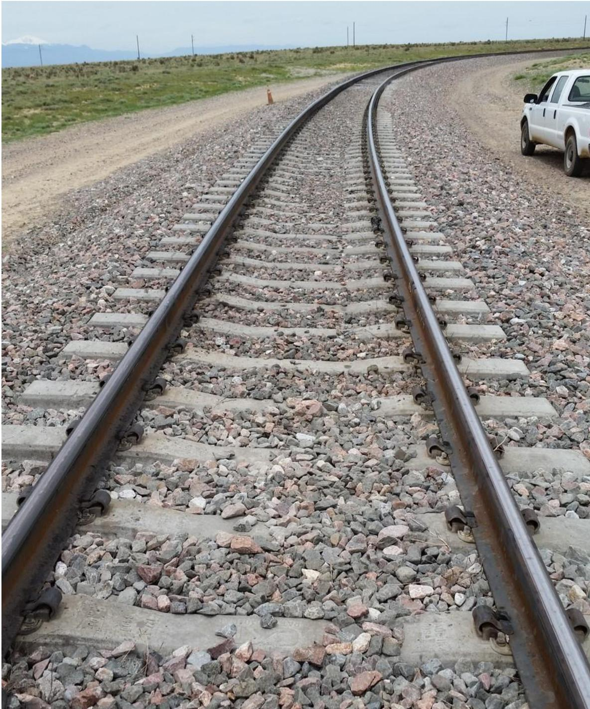
Figure 127 “T”-marked crossies installed in curved track during Stage III
