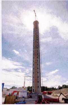
ThyssenKrupp test tower.
