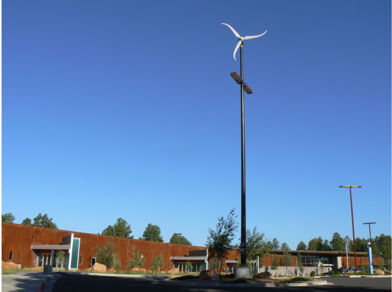
Figure 1.3 Example of the a Skystream wind turbine installed at Coconino Community College. [Photo Courtesy of [6]]
