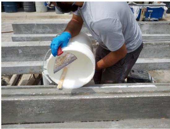
Figure 3-18: Procedure of Applying Epoxy Into the Grooves.
