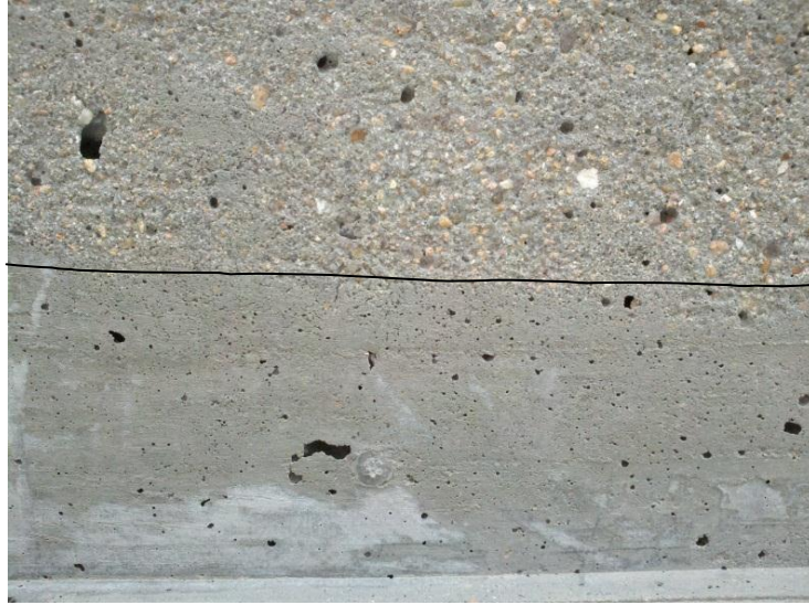
Figure 3-21: In the Top is Sandblasted Surface; In the Bottom is Unsandblasted Surface.
