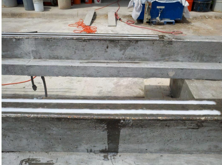
Figure 3-19: NSM Bars inside the Grooves Covered with Epoxy.
