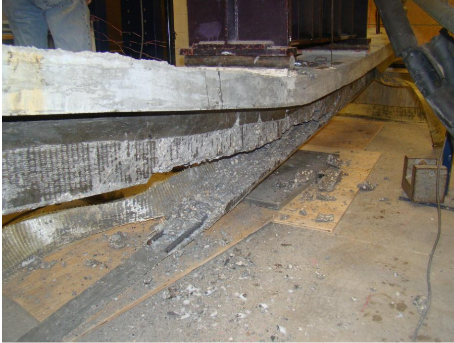
Figure 4-24: Premature Failure Due to Stresses Concentrations at the End of the Rebar in Beam T4.
