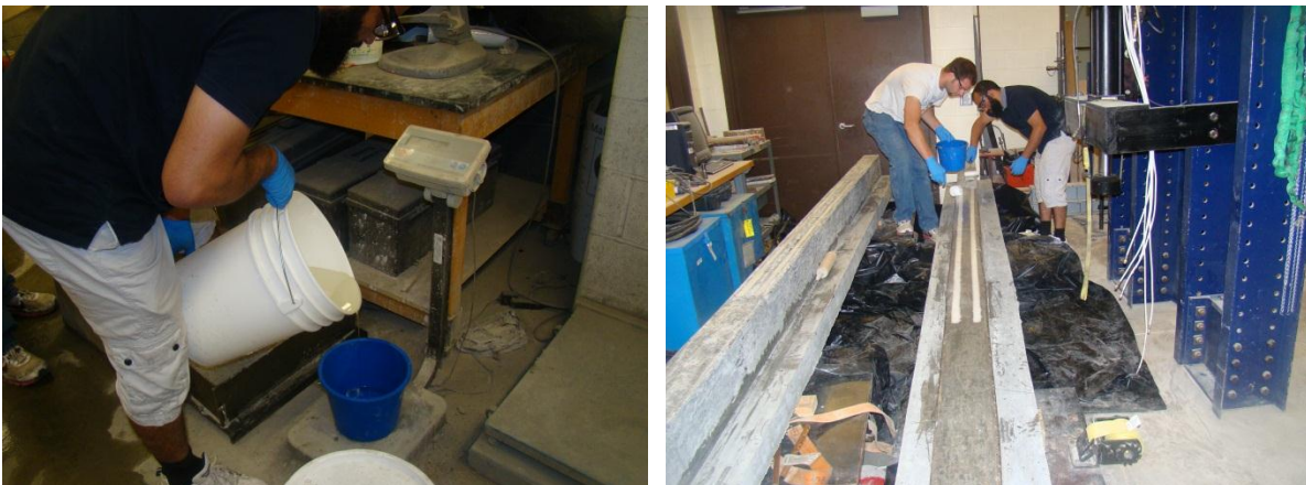
Figure 3-22: Epoxy Mix and Applying Procedure.
