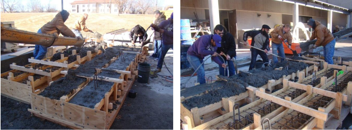
Figure 3-2: Casting of the Concrete T-Specimens.
