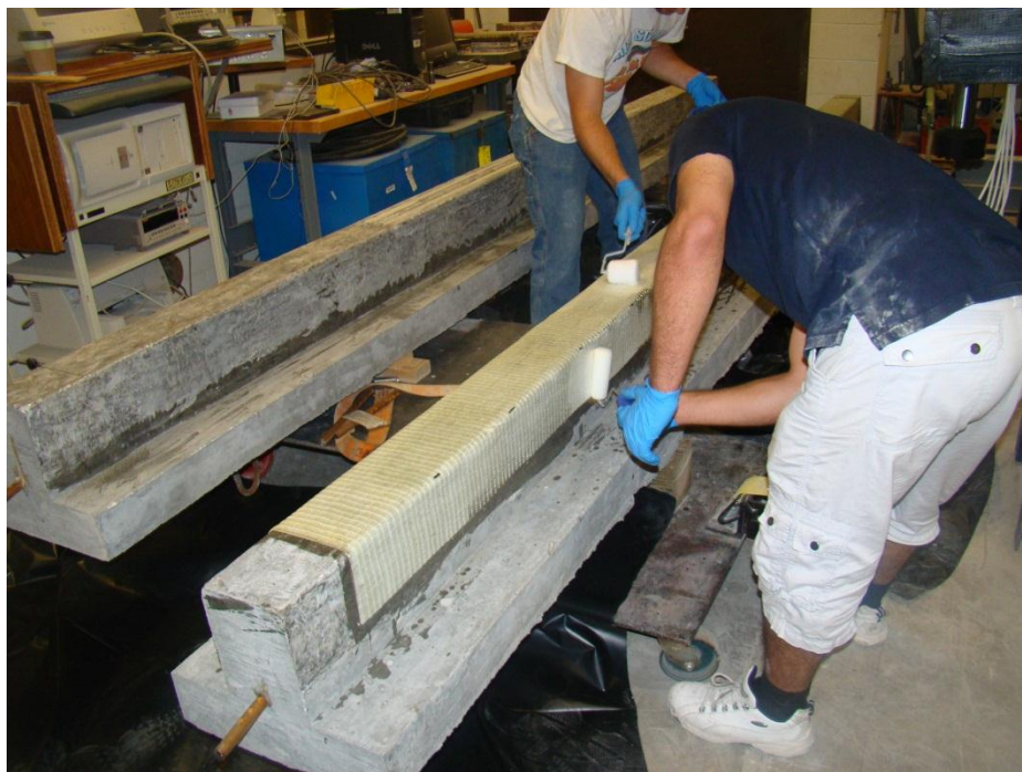
Figure 3-24: Applying the Epoxy Resin Coating with the Roller.
