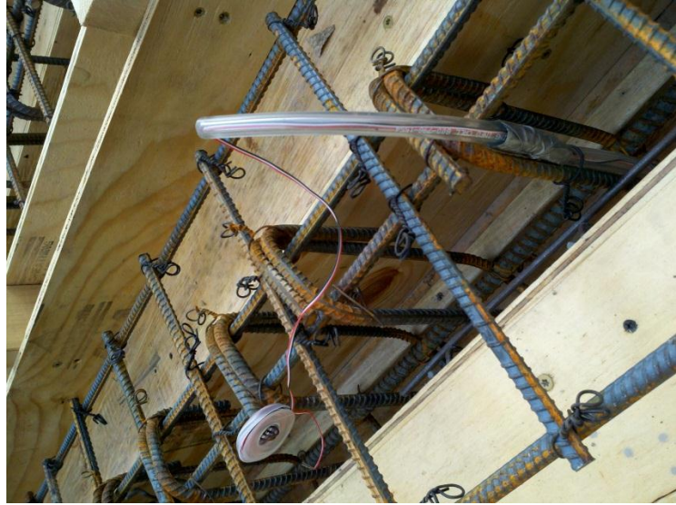
Figure 3-15: The Strain Gage Wire Protected by a Plastic Hose.
