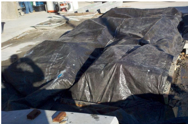
Figure 3-3: Curing of the Concrete by Covering with Plastic Blanket.
