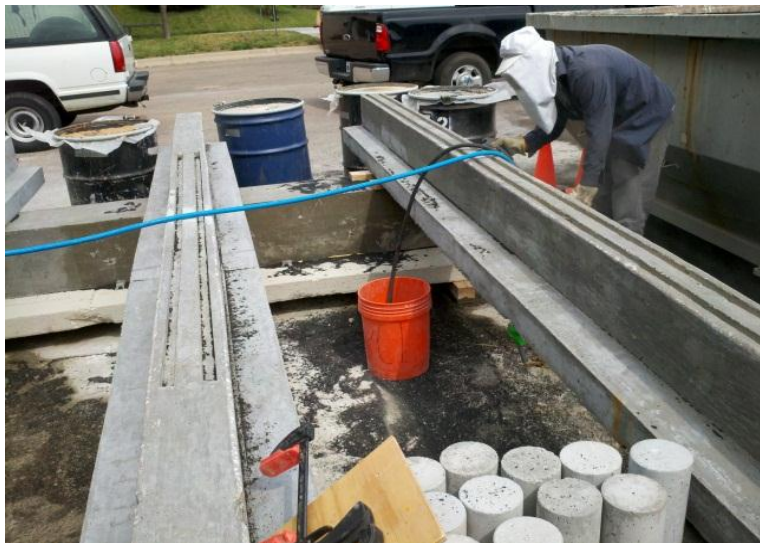
Figure 3-20 : Beam Sandblasting Process.
