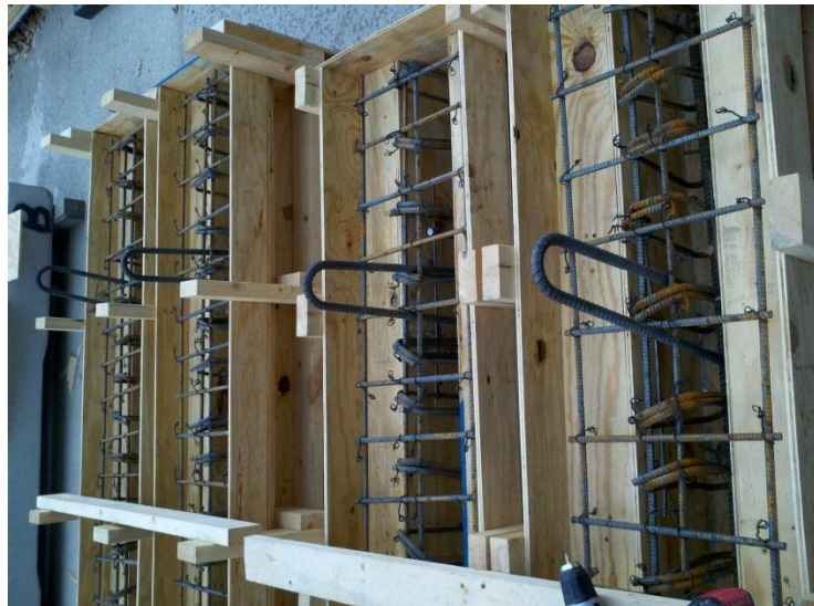
Figure 3-16: The Rebar Cages Inserted Into the Formwork and Prepared for Casting.
