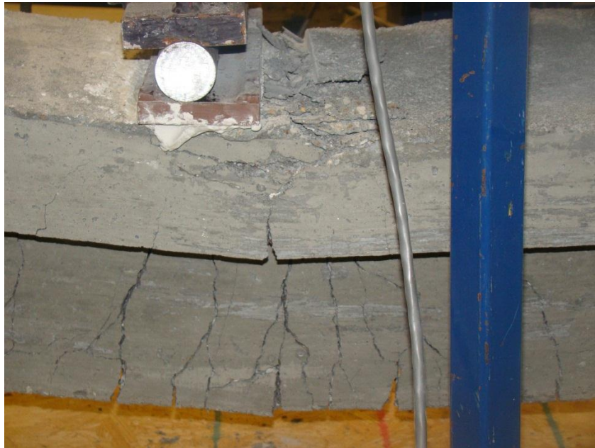
Figure 4-3: Beam T1 after Concrete Crushing Failure.
