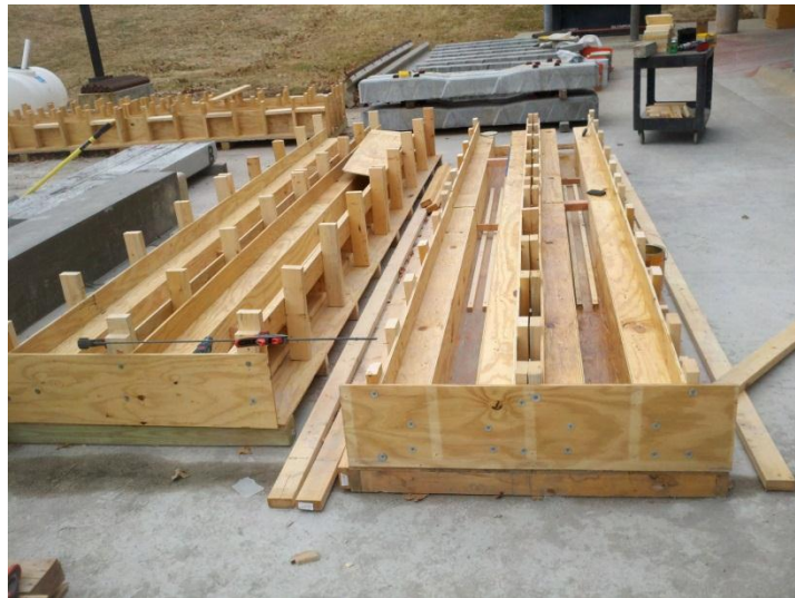
Figure 3-11: Top view of the Formwork Place for T-Specimen Casting.
