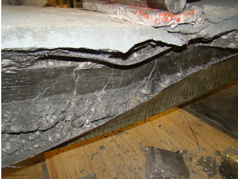
Figure 4-9: Shows the Yielding of Compression Steel at the Flange of Beam T2.
