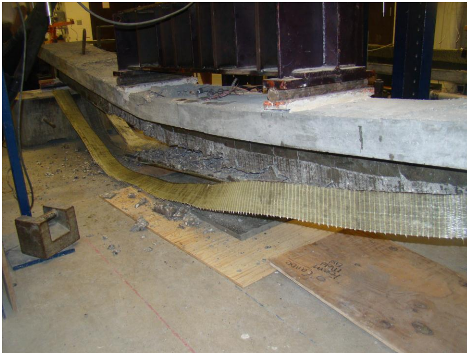
Figure 4-25: Premature Cover Delamination Failure Followed with GFRP Debonding of Beam T4.
