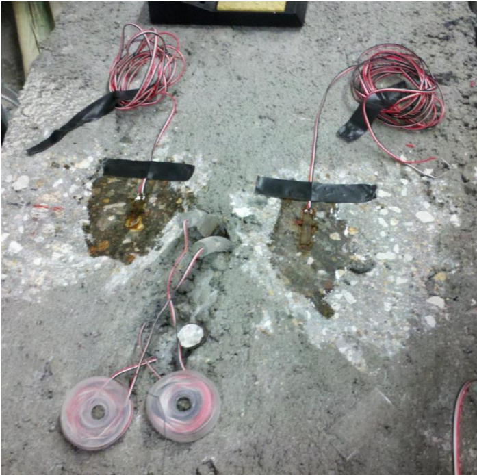
Figure 3-29: Two Strain Gages at Concrete Upper Face.
