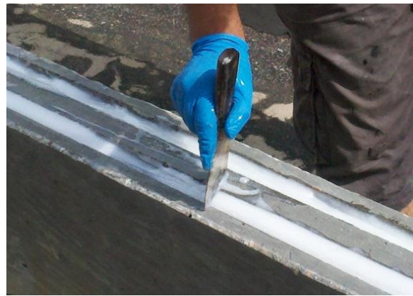
Figure 3-18: Procedure of Applying Epoxy Into the Grooves.
