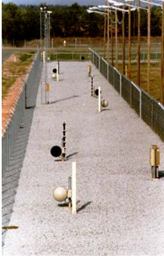
FIGURE 2. Clear zone with multiple sensors – part of a robust security system that is not appropriate for the carcass disposal operations problem.
