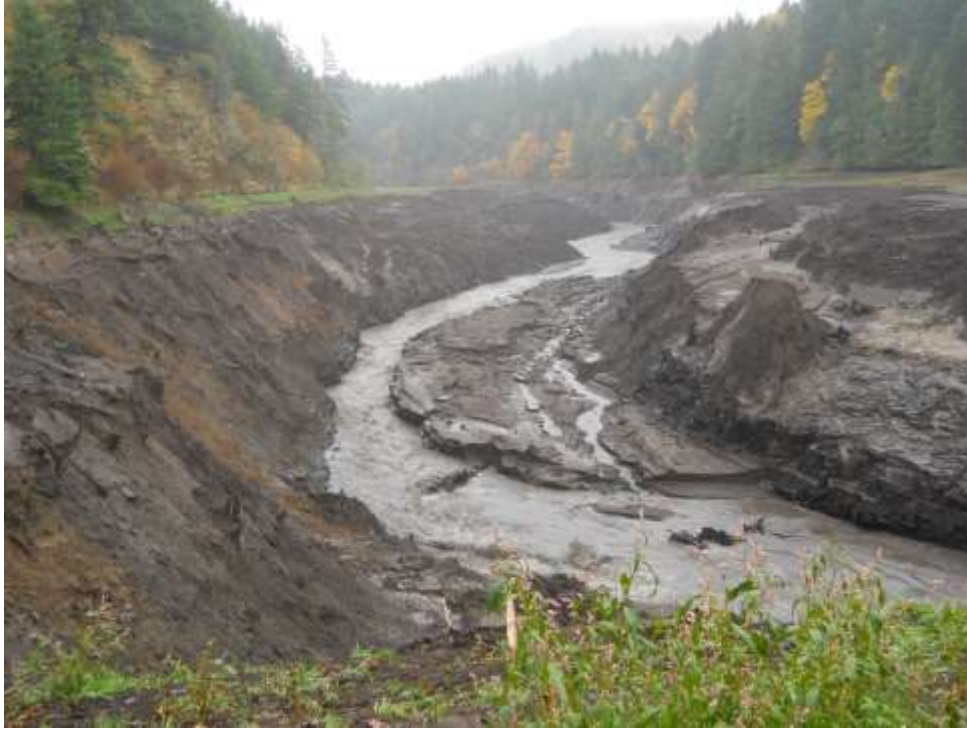
Figure 3.17. Northwestern Lake draining following Condit Dam removal, October 30, 2011 (photo courtesy of Wayne Lease).
