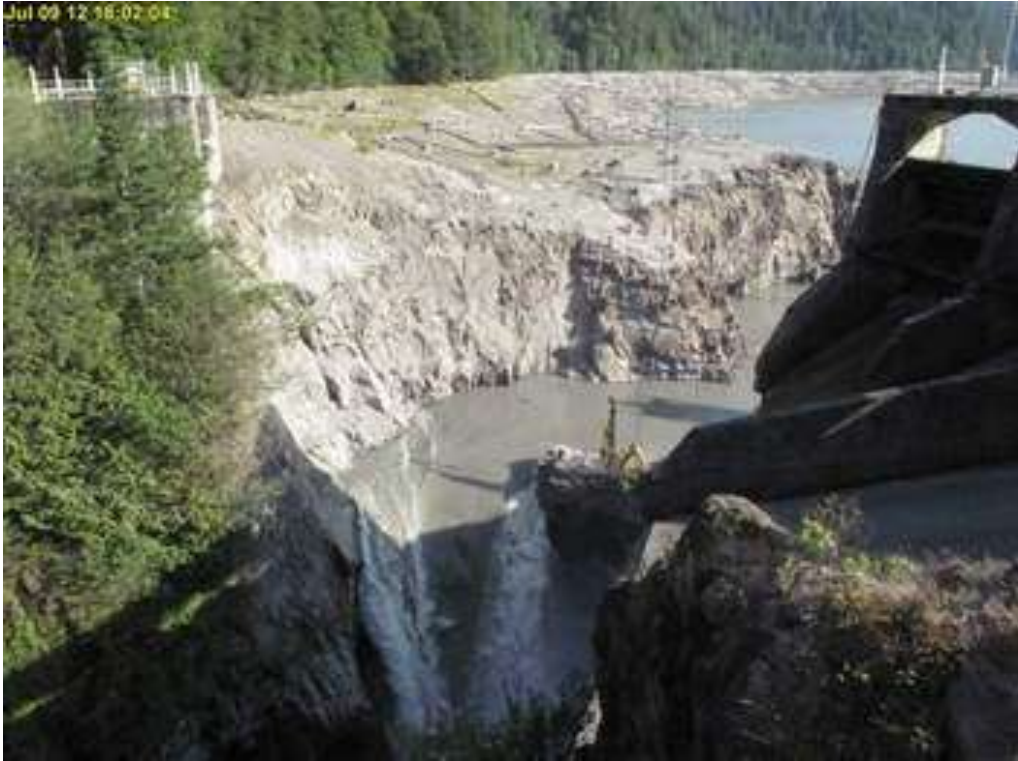
Figure 3.8. Glines Canyon Dam removal in progress, 9 July 2012 (Peninsula Daily News 2012).
