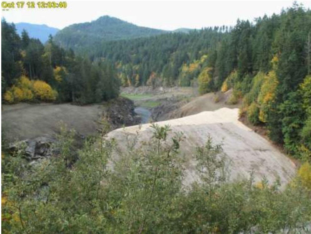
Figure 3.10. Lake Aldwell (Elwha Dam) finished draining (Photo: Erdman Video Systems, Inc. 2013).
