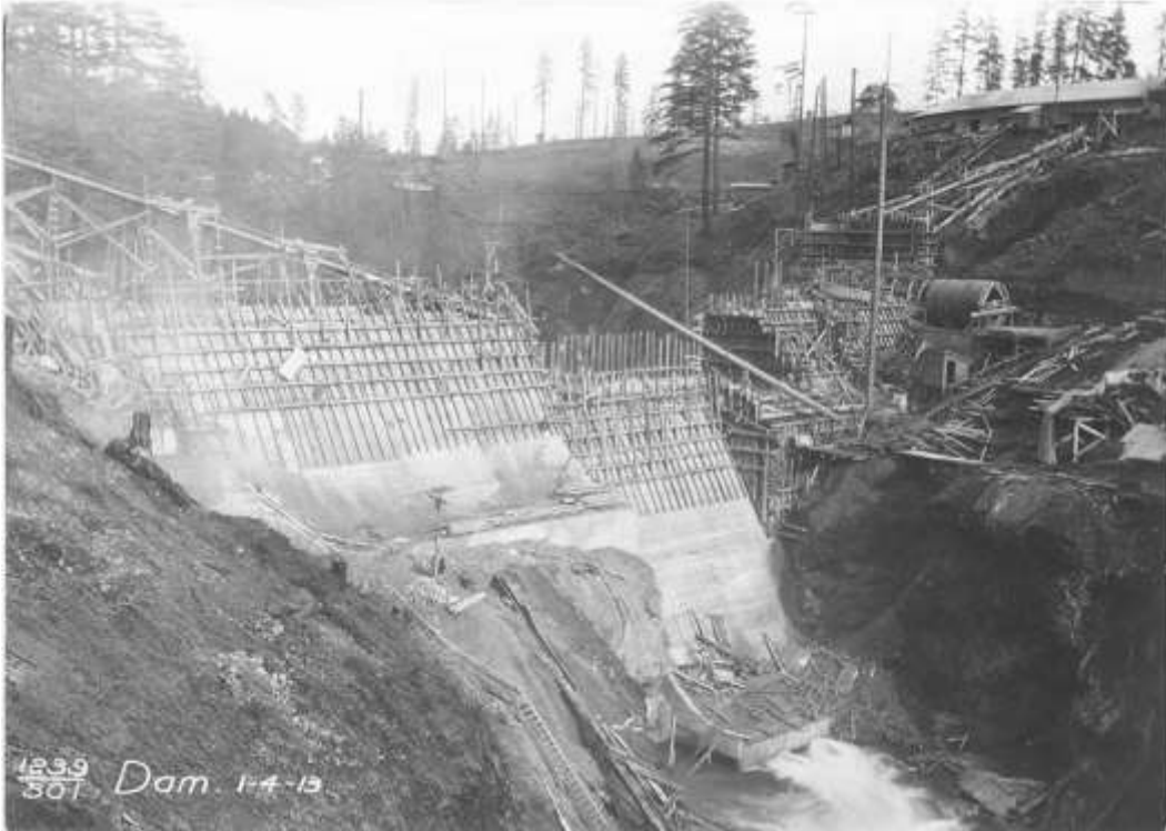
Figure 3.15. Condit Dam, construction, January 1913 (source: PacifiCorp 2013)
