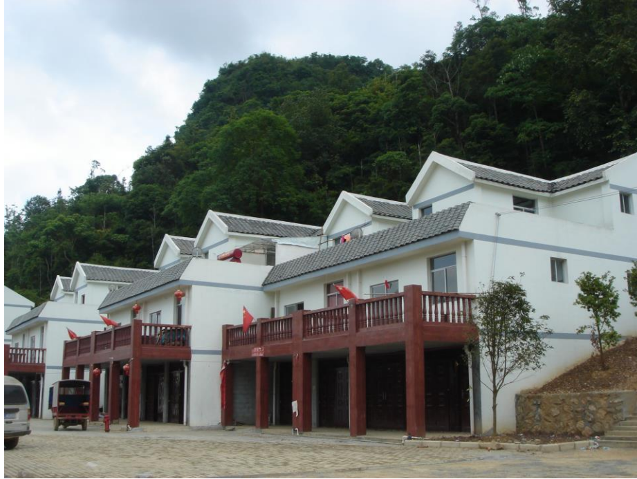
Figure 5.6 Border Houses in Longbang, Jingxi, China. Front. June. 2011. LongBang Town, Guangxi, China. Photo: Lianling Su
