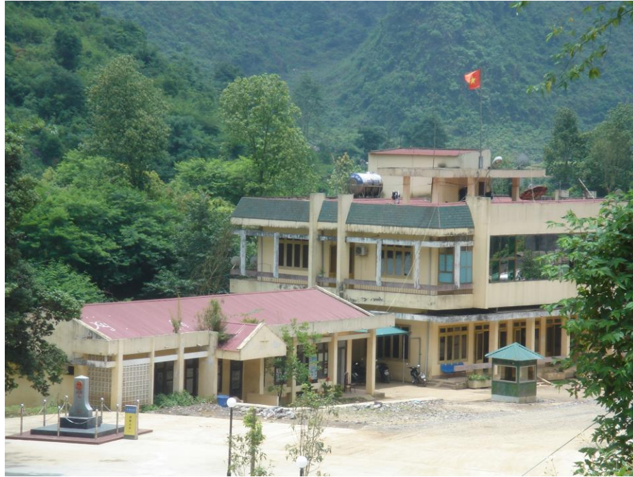
Figure 3.4 The Official Border Checkpoint in Cao Bang ,Vietnam. June 2011. (Photo was Taken from Longbang, Guangxi, China.) Photo: Lianling Su
