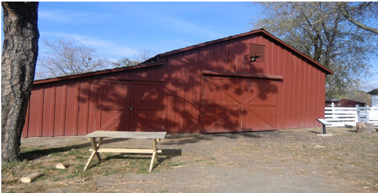
Figure 3. Photograph of the slightly restored Mahaffie barn as it appeared in October, 2012. Photograph by author. The farm side of business would play a vast role when dealing with storage and providing resources for themselves and their people they supplied to.
