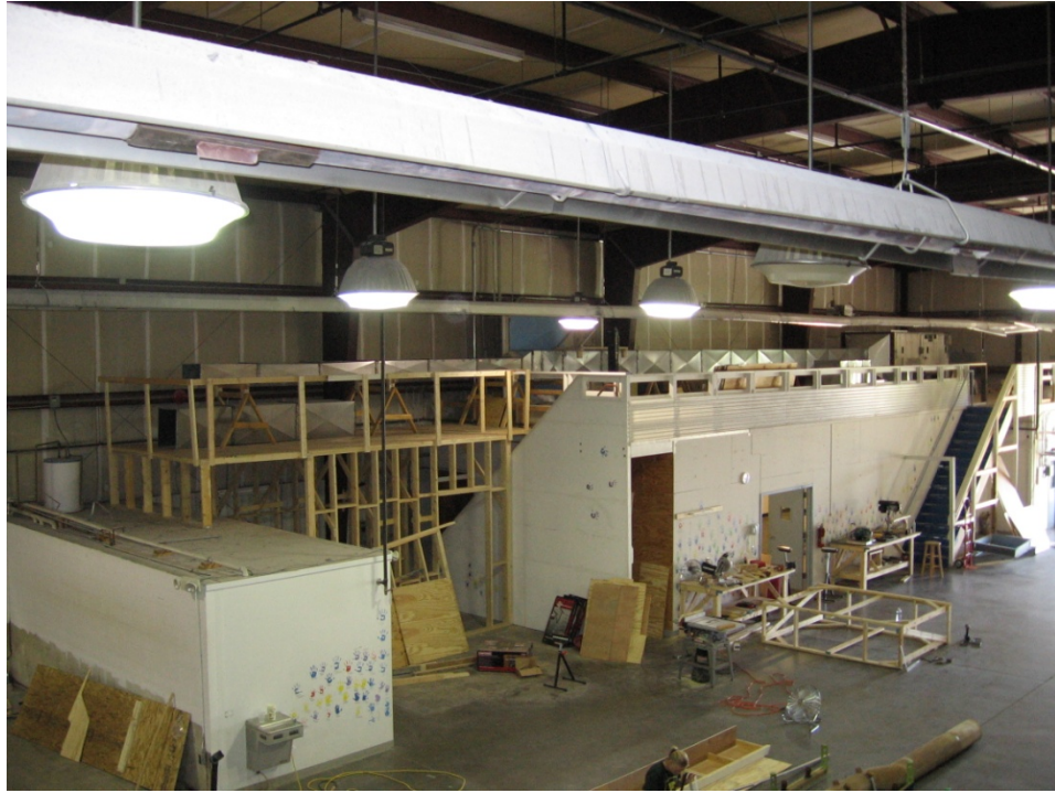
Figure 2.3 General Test Site 1
