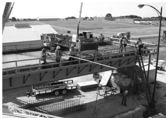
Fig. 3—Bridge during deck placement.
