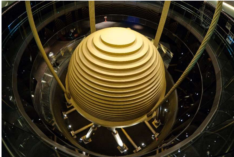
Figure 18 Picture of Taipei 101 TMD (Photograph from Plessis, 2010)
