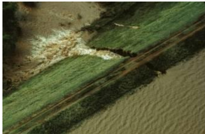
Figure 1.1 Internal Erosion Event, Upper Red Rock
