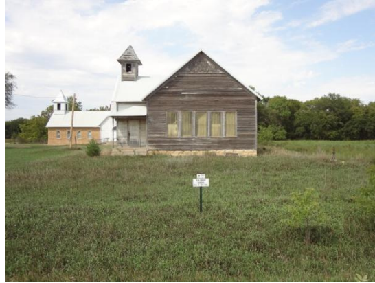
Figure 15. Photograph of Ash Grove School Fall 2012 Taken by Author
