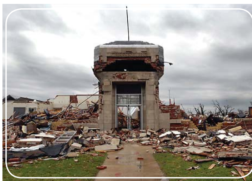
Figure 7.2 Greensburg's school following the disaster
