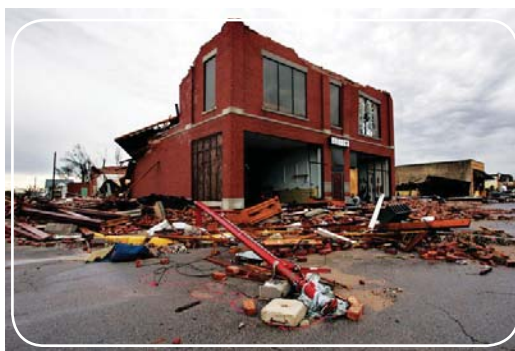
Figure 7.3 Remnants of Greensburg's downtown
