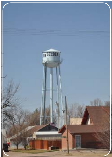
Figure 4.62 Selden Water Tower
