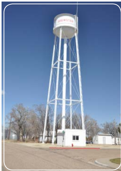
Figure 4.63 Brewster Water Tower
