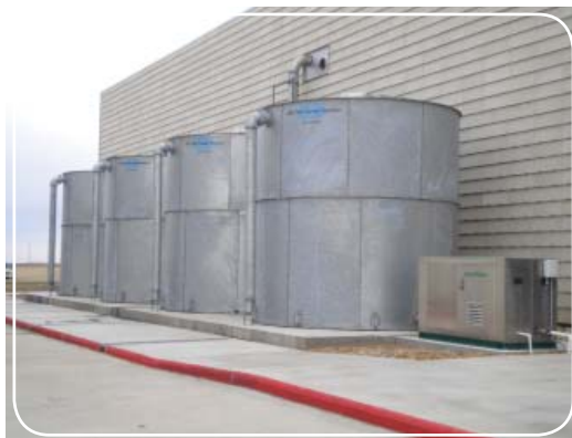
Figure 4.44 Runoff storage cisterns at High School
