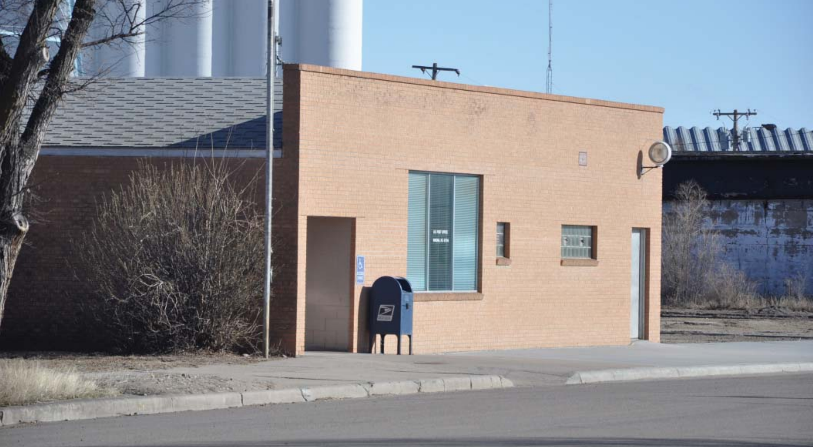
Figure 5.14 Post Office entry - existing condition
