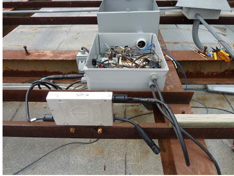
Figure 6-4 Enphase M190 Installation Photo
