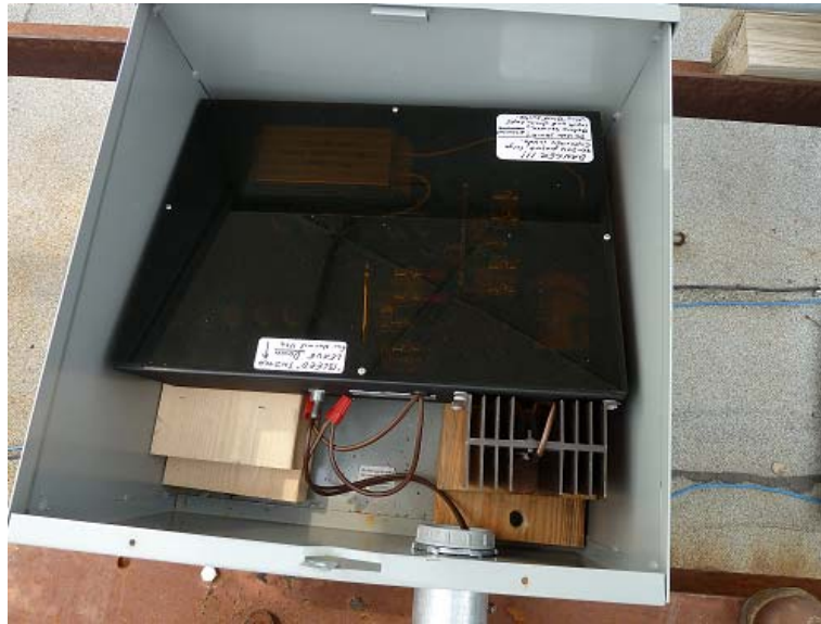
Figure 6-8 Capacitor Box Installation Photograph
