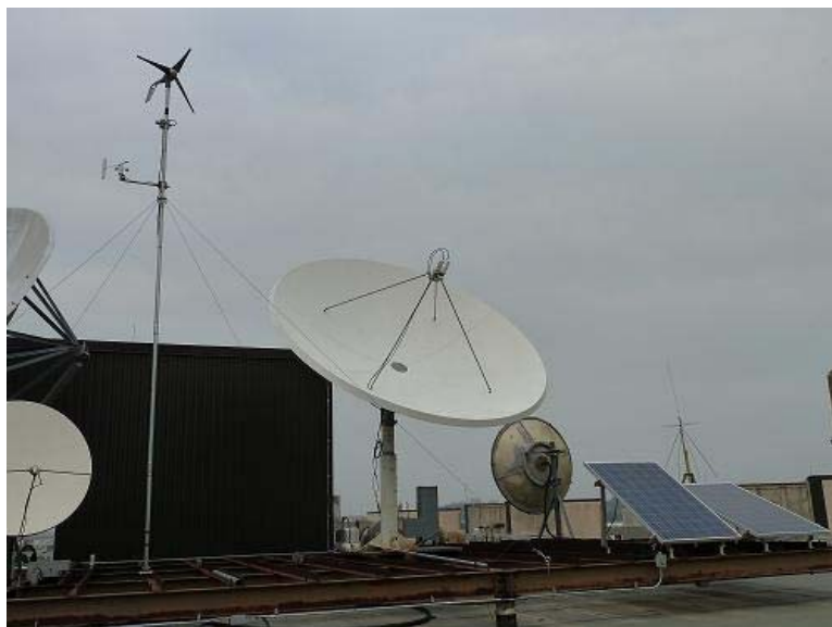
Figure 1-1 Rathbone Rooftop Installation Photo
