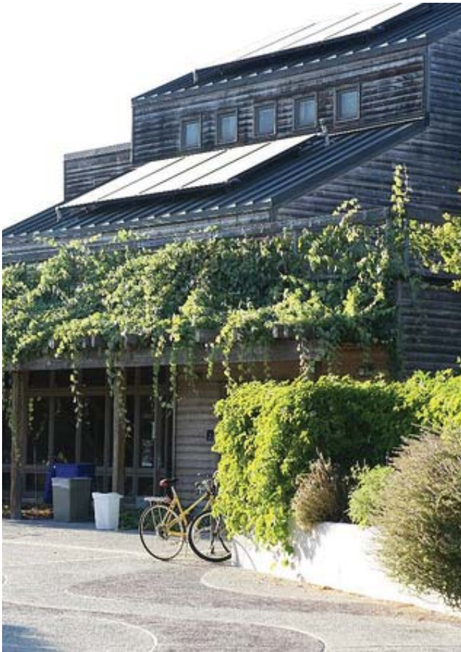
figure 4.29 A southern trellis provides shade
