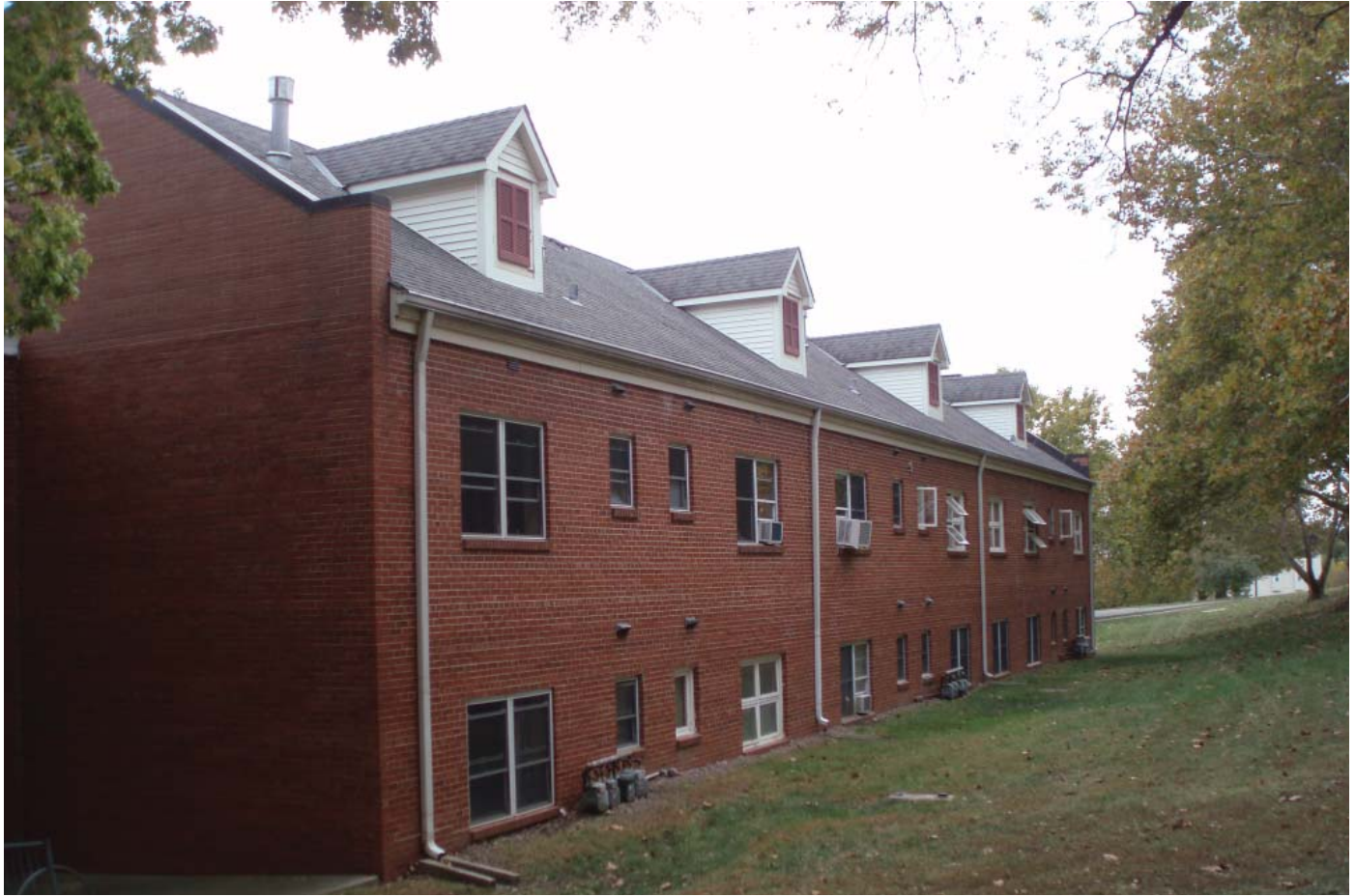
figure 5.15 View of building rear
