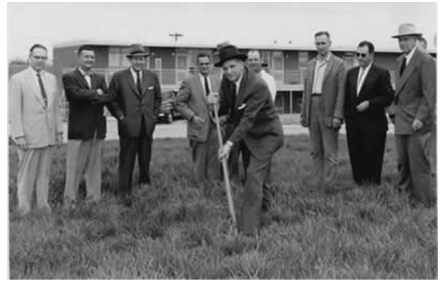
figure 4.6 Ground-breaking of a 1950's building
