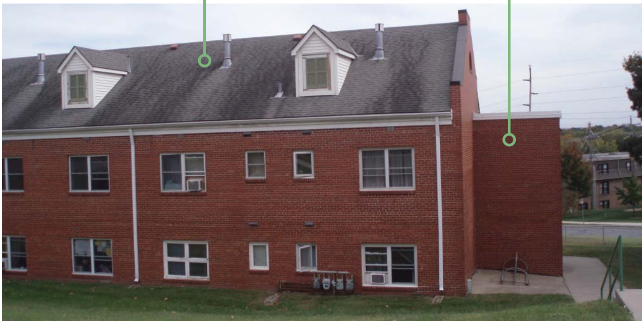
figure 5.20 View of building roof
