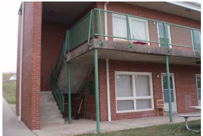
figure 5.17 Typical building stairwell
