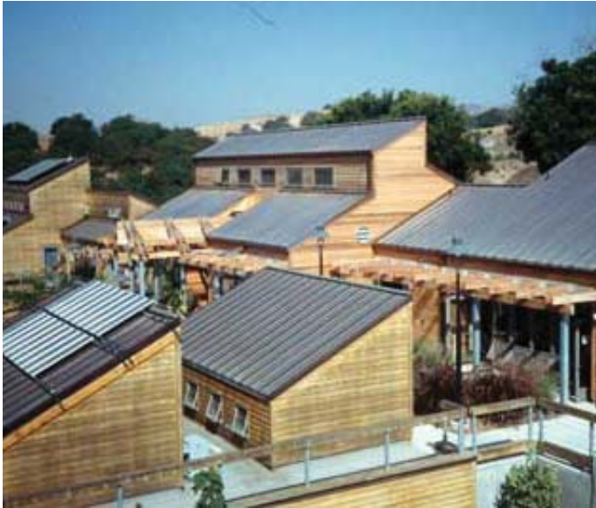
figure 4.36 Roof-mounted solar collectors
