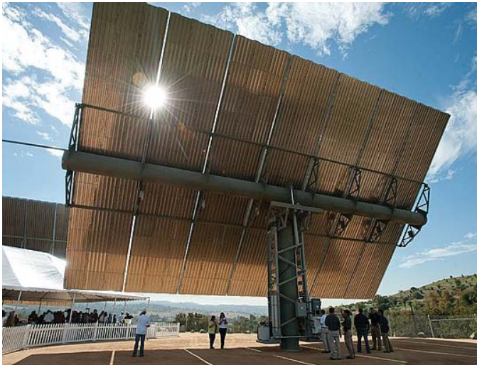
figure 4.38 Solar tracking photovoltaics
