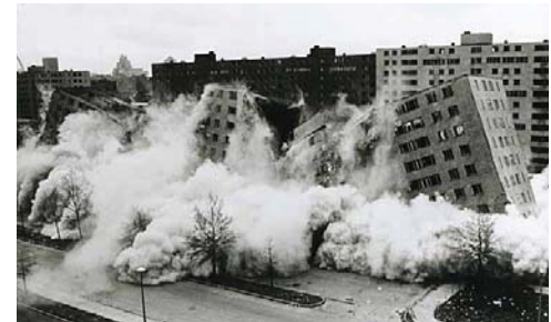
Figure 1.2: Image of Pruitt-Igoe Demolition. Photo from ( www.so-and.org ).
