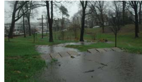
Figure 3.24: Image of Stormwater BMPs. Photo from ( www.wordpress.com ).
