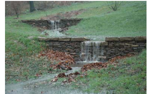
Figure 3.22: Image of Stormwater BMPs. Photo from ( www.wordpress.com ).
