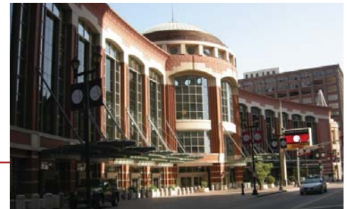
Figure 1.10: Image of the America's Center Convention Complex. Photo by Author.
