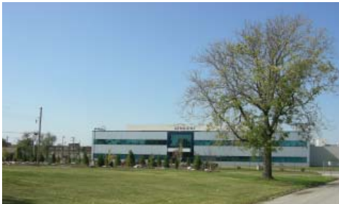
Figure 4.27: Industrial Site. Photo by Author.
