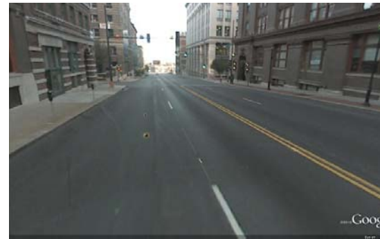
South Broadway Boulevard Kansas City, Missouri (Google Street View)
