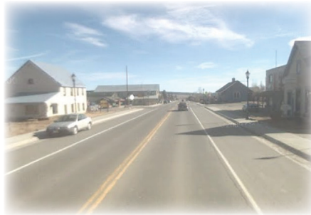
figure 4.5 poorly defined Main Street (adapted from: Google 2010)
