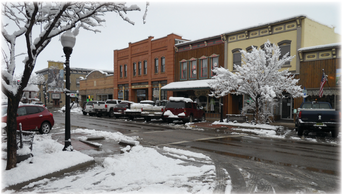
figure 5.85 3rd street existing conditions (murner 2011)
