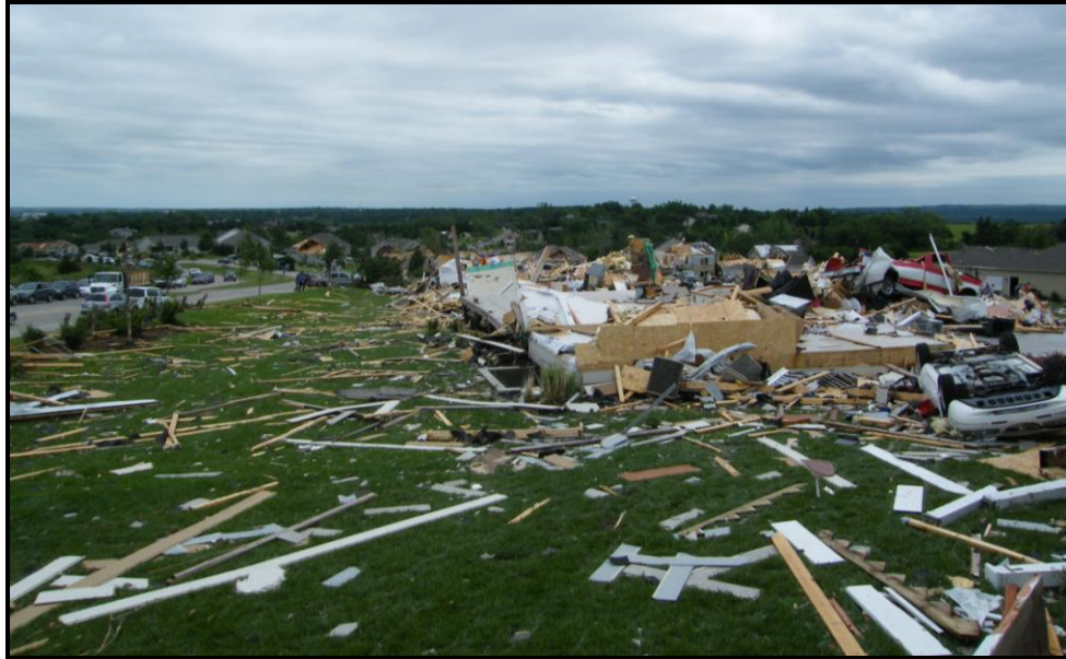
Figure 4.26: EF-4 damage in the Amherst residential area, Manhattan, KS (photo by author, taken with homeowner's permission, on 12 June 2008; the morning after the tornado).
