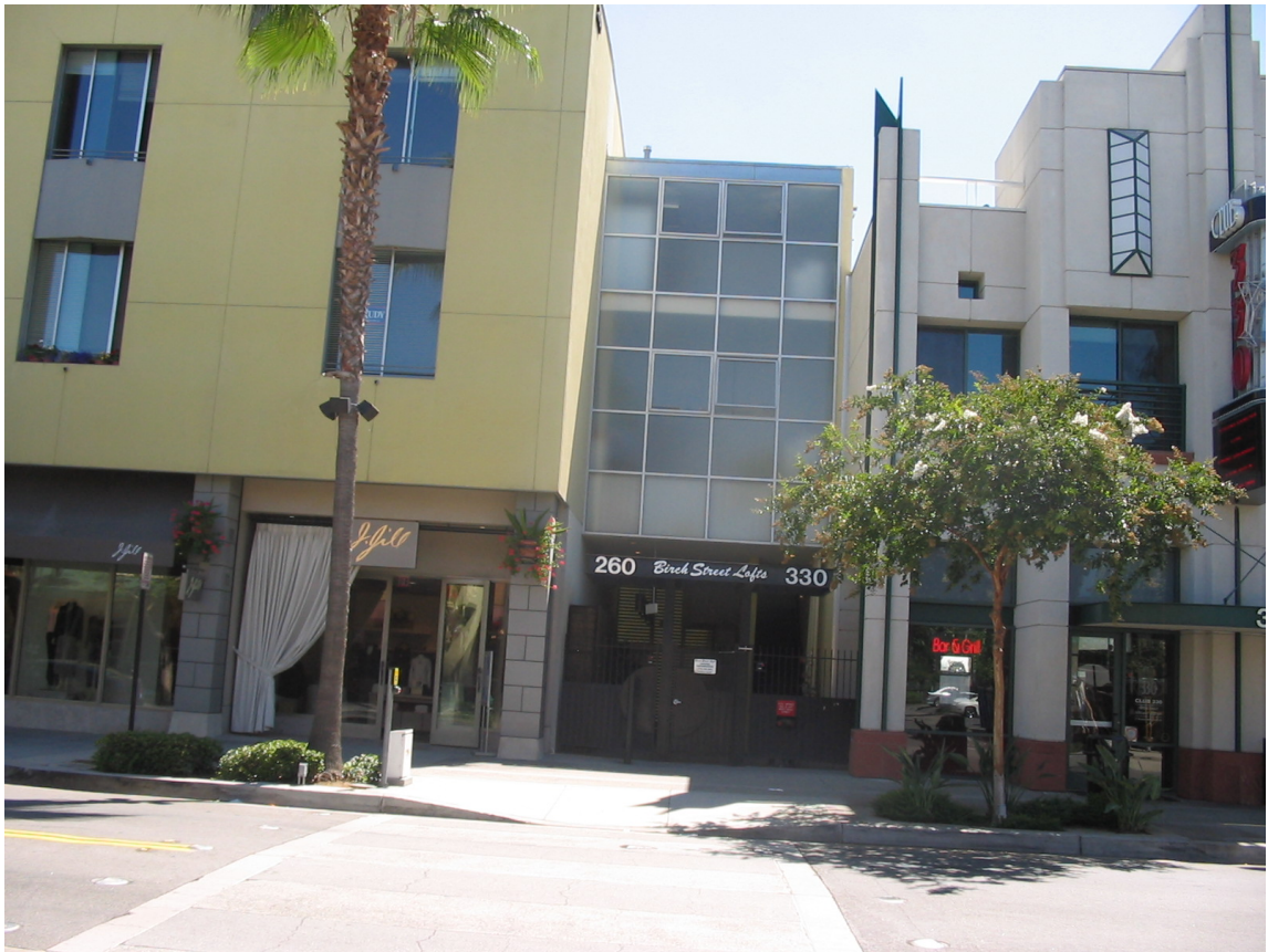
Figure 6.1 Entrance to the Birch Street Lofts, (Antonini, 2007)
