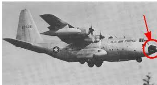
Figure 2-1 WWII Aircraft FRP Radome
