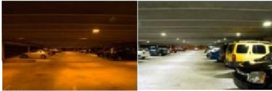
Raleigh, NC Parking Garage before with HPS lamps
