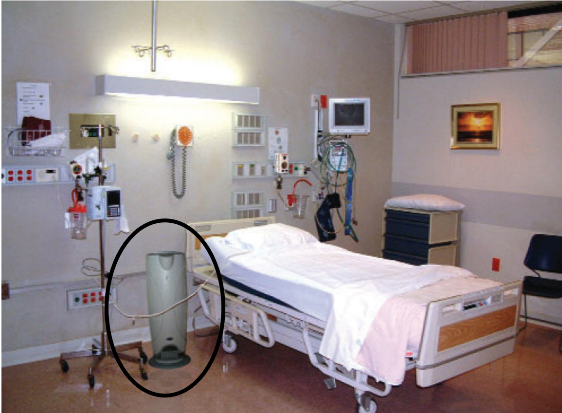
Figure 4.11 Portable UVGI Unit with Fan (W. J. Kowalski, 2007)
