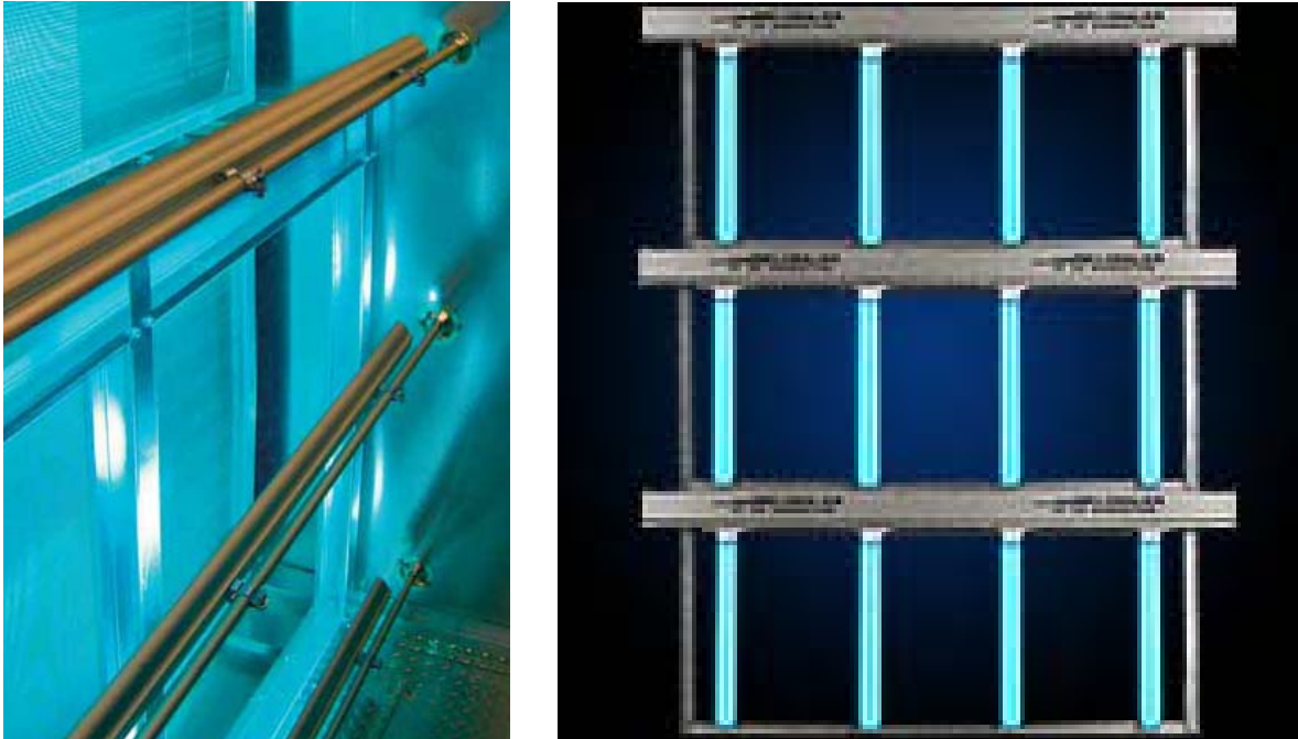
Figure 4.3 UVGI Lamp Systems in AHU: Horizontal and Vertical
