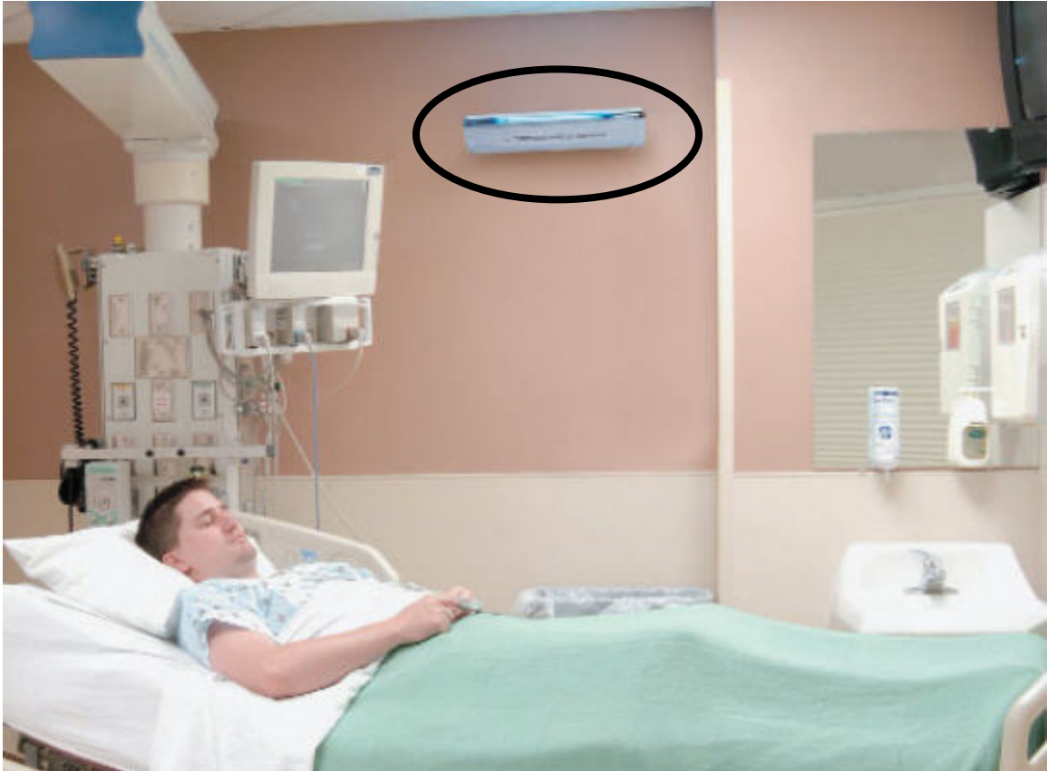
Figure 4.10 Upper-Room UVGI Installation
