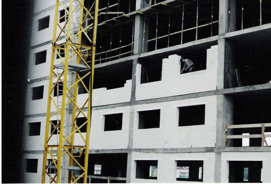
Figure 4.1: AAC used as an exterior non-bearing wall in Warsaw, Poland (Stephens)
