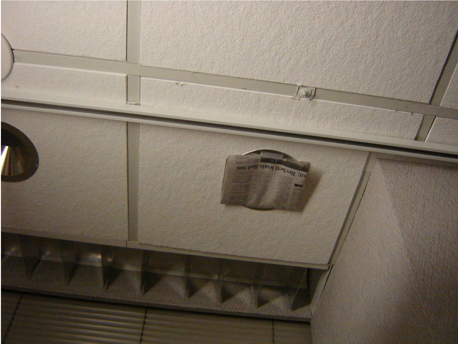
Figure C.8 Typical Obscuration Method for Undesired Fixtures
