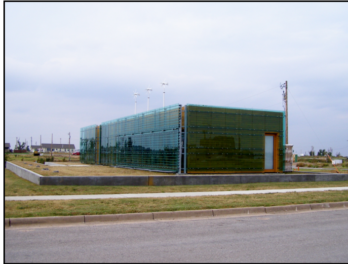
Figure 4.8 LEED Platinum 5.4.7 Arts Center in Greensburg, Kansas. Photo by author.
