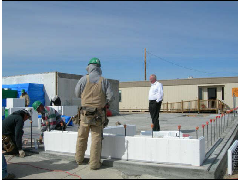
Figure 4.11 ICFs used to form walls of Greensburg State Bank. Photo courtesy of Dea Anne Corns.
