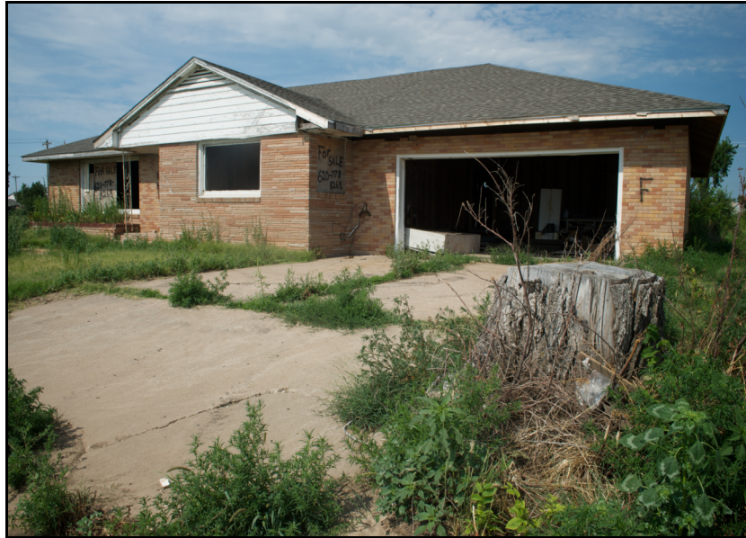
Figure 4.16 Unkept, Damaged House in Greensburg. Photo by author.
