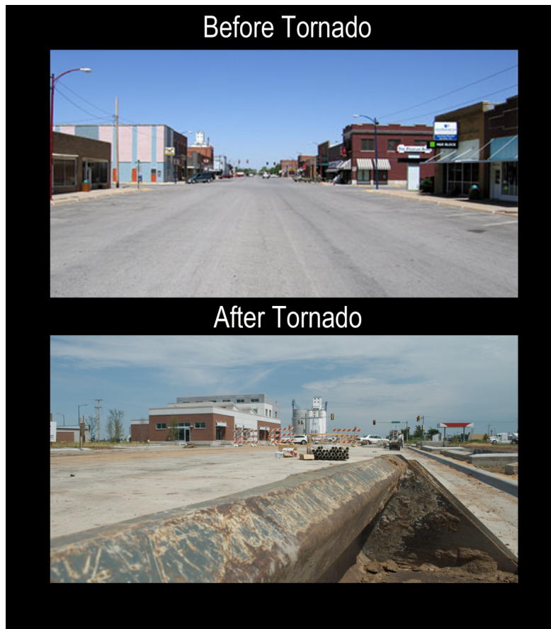
Figure 4.15 Green streetscape under construction after the May 4, 2007, tornado. Top photo courtesy of J. Schumacher. Bottom photo by author.
