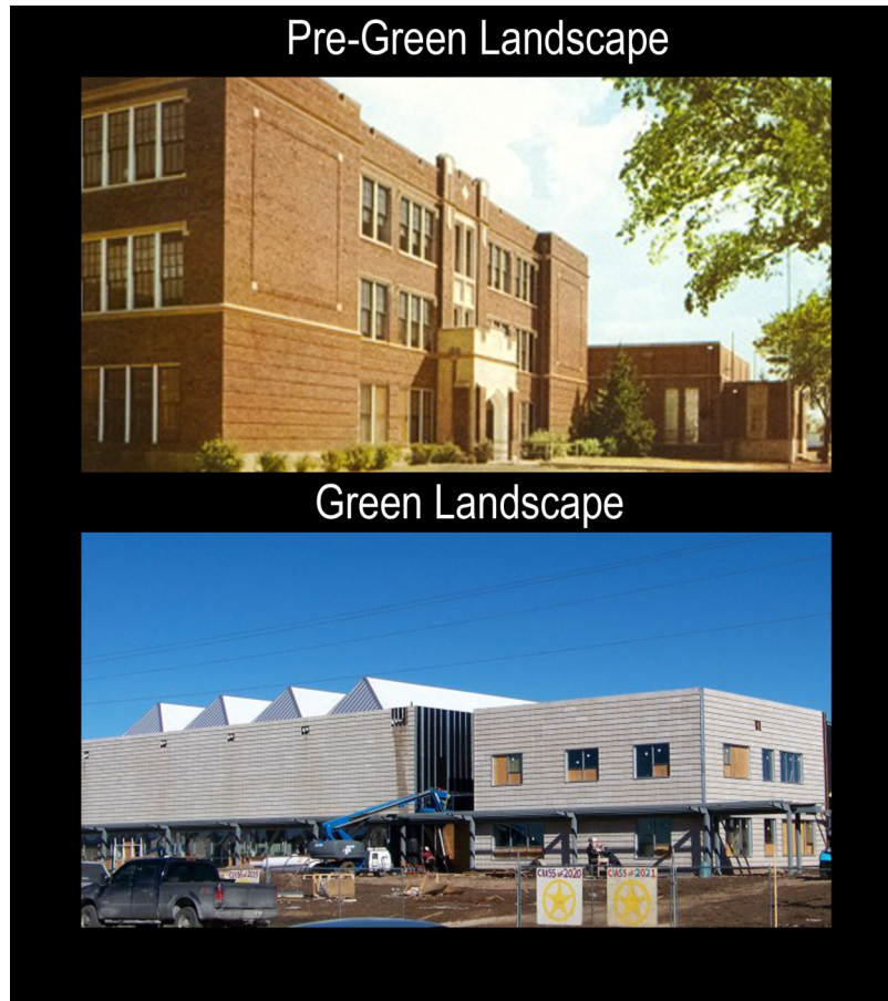
Figure 4.12 Greensburg's new, Green, school under construction. Top photo courtesy of Cheryl Richard. Bottom photo courtesy of USD 422 website.
