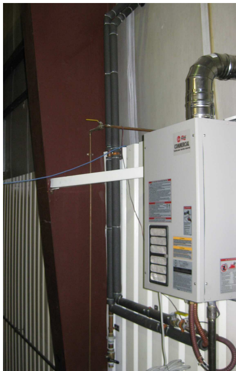
Figure 2.16: Heating Loop Water Heater
