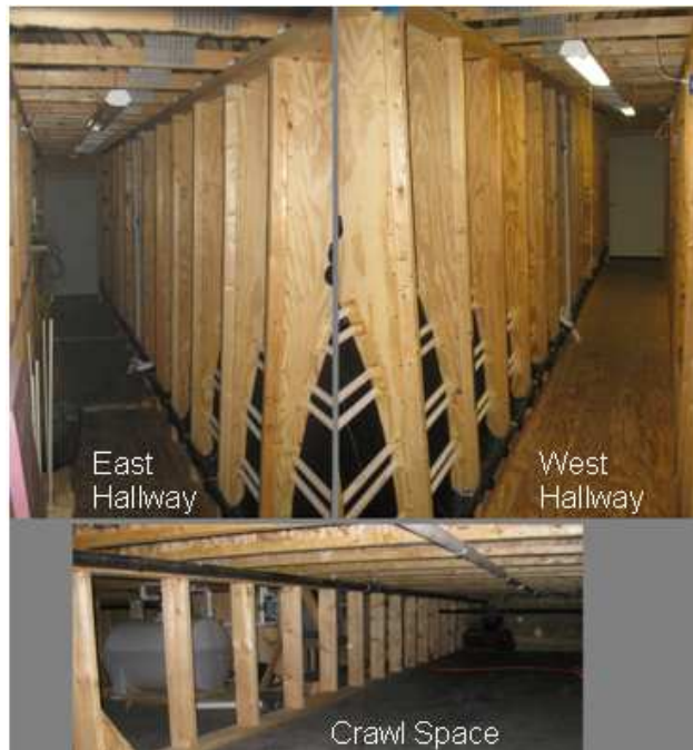
Figure 2.2: Chamber Hallways and Crawl Space
