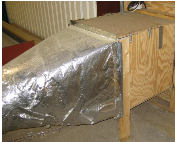
Figure 2.18: Inlet Filter Housing
