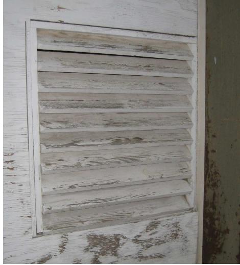
Figure 2.19: Supply Air Louvered Inlet
