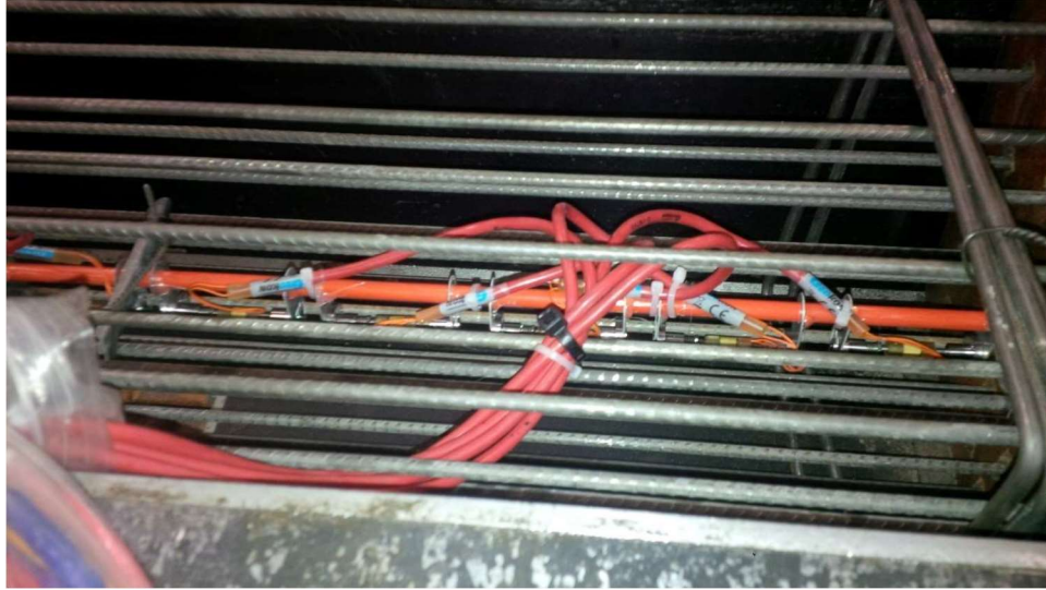
Figure 3.4 VWSG installed at center of a Nortrak tie
