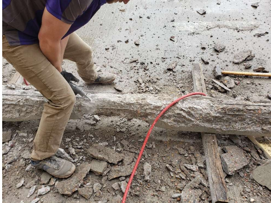
Figure 7.9 Extraction of wires from tie
