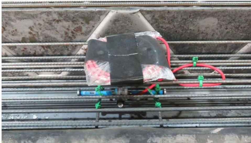
Figure 3.3 VWSG installed at center of a Rocla tie
