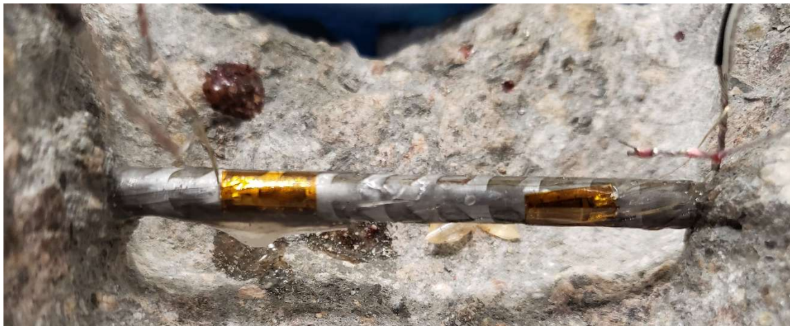
Figure 6.11 Close up of gages 1 and 2 on tie NT-1
