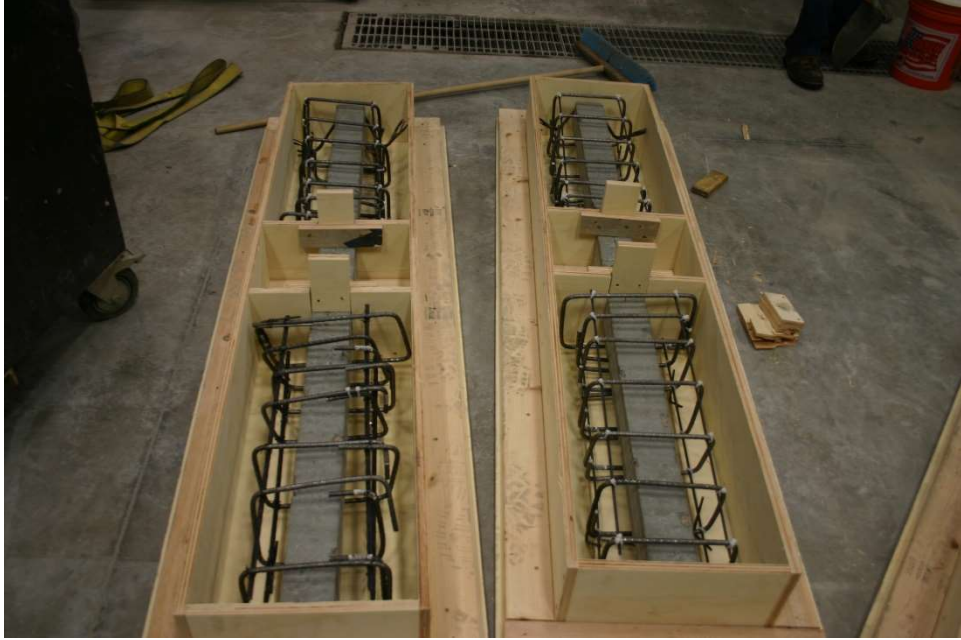
Figure 5.5 Prisms with rebar cages prior to casting blocks
