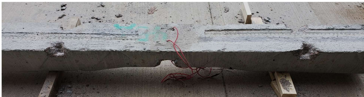
Figure 7.17 Wired exposed on tie for marking 60 inch gage length
