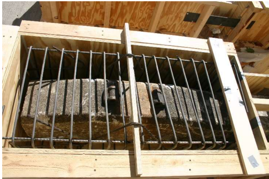
Figure 5.24 Typical rebar cage
