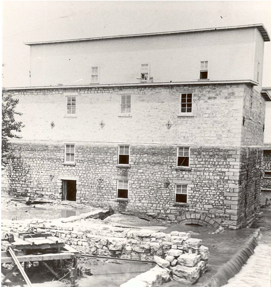
Figure 4. General Samuel Wardens Mill in the Southern territory of Marshall County, along the West bank of the Big Blue River, Township of Irving, Circa 1870 Marshall County Museum and Historical Society.
