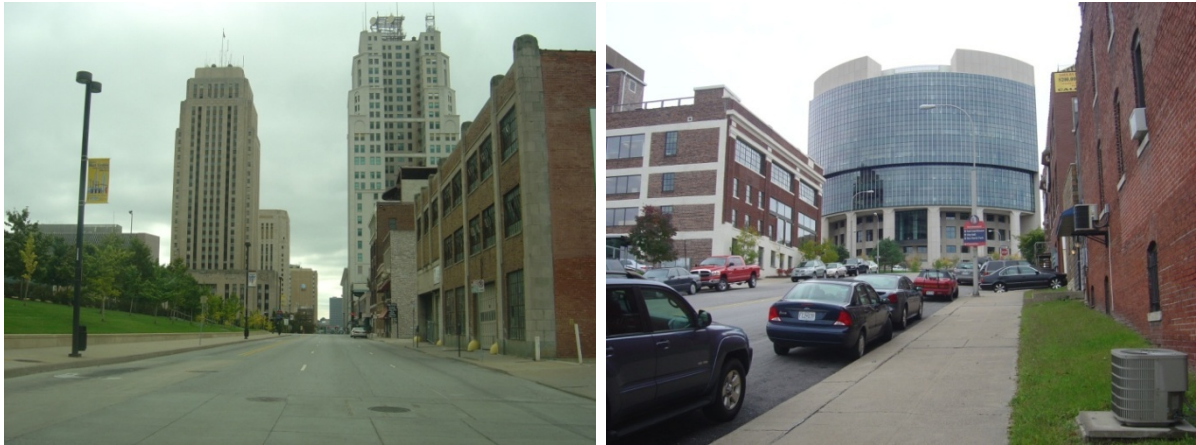
Figure 3-9. City Hall (left) and US Courthouse (right) in Government District. (Source: Photograph by author).
