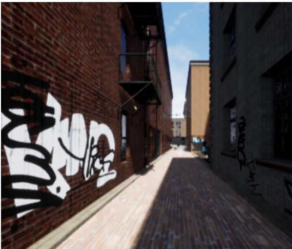
Figure. 3.7. Unmaintained buildings. Building Maintenance variable level 2 (unmaintained building facades).
