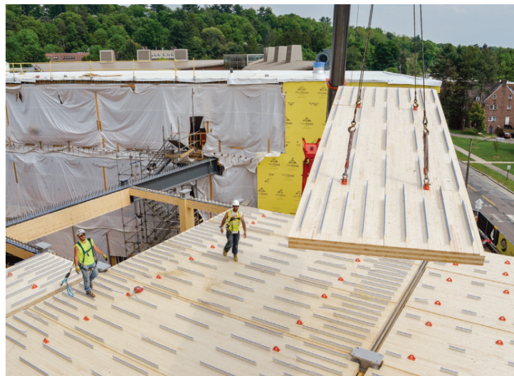
Figure 5-1: Installation of CLT Panels (Lathe, 2017)
