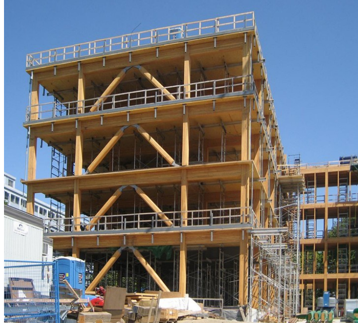
Figure 5-2: Installation of CLT floor with HBV shear connectors (ThinkWood, 2012) LifeCycle Tower One
