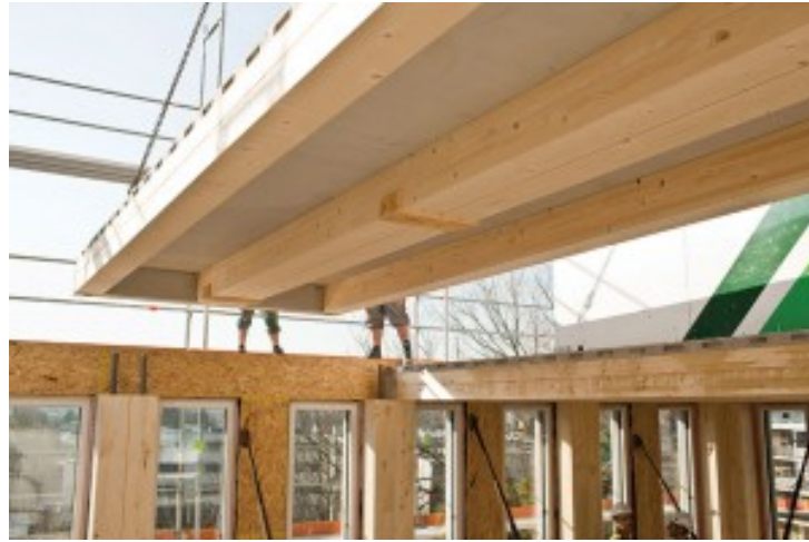
Figure 5-3: Installation of prefabricated TCC floor
