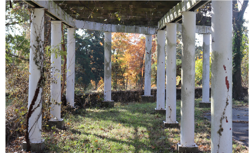
Figure 2.10: Osawatomie State Hospital.
