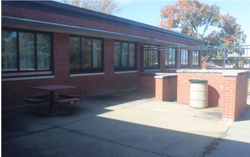
Figure 2.9: Osawatomie State Hospital.
