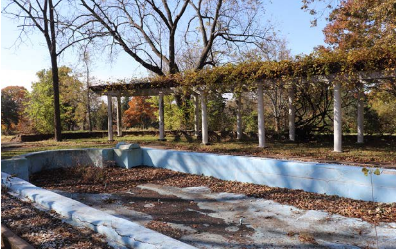
Figure 2.17: Osawatomie State Hospital.
