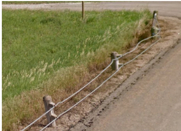
Figure 218: Low-Tension Cable Guardrail
