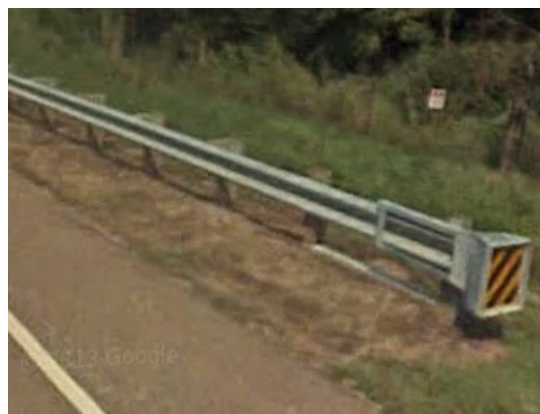
Figure 28.15: Energy-Absorbing Guardrail End in the Field
