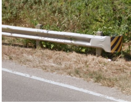
Figure 29.16: Breakaway Cable Terminal in the Field
