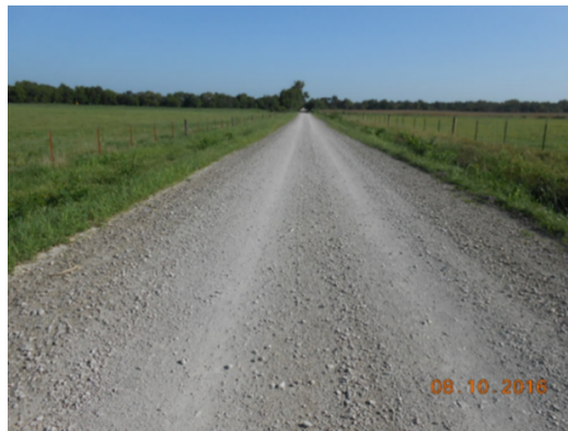
Figure 35.22: Rural Two-Wheel-Track Gravel Road (Bowers, 2019)
