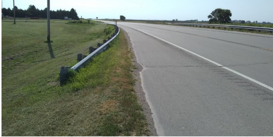
Figure 43.30: Guardrail Shielding a Culvert (Bowers, 2019)
