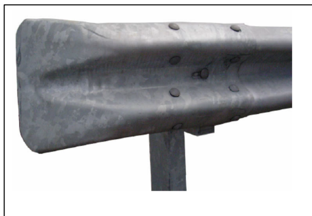
Figure 1.3: Blunt-End of Guardrail (Glennon & Engr., 2012)
