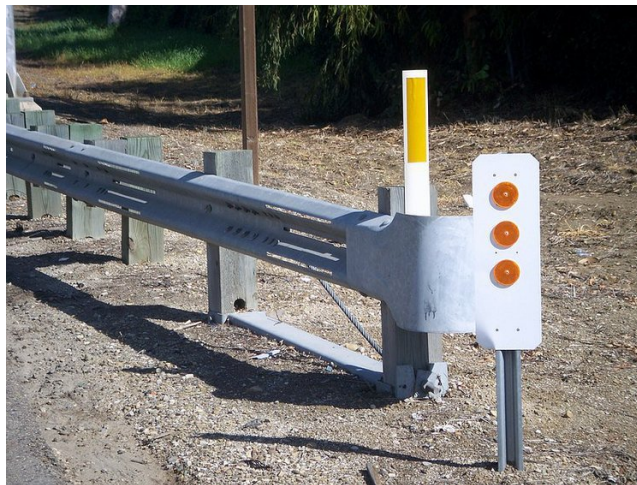
Figure 1.6: Breakaway Cable Terminal
