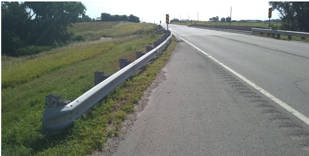
Figure 50.37: Bridge-approach guardrails to Bridge End (Bowers, 2019)
