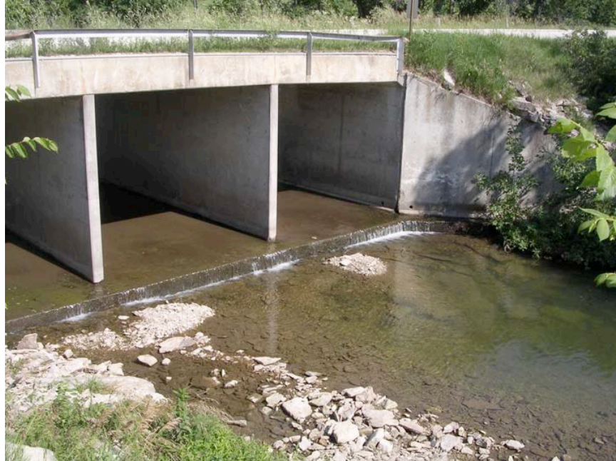
Figure 41.28: Culvert on Rural Road (Bowers, 2019)
