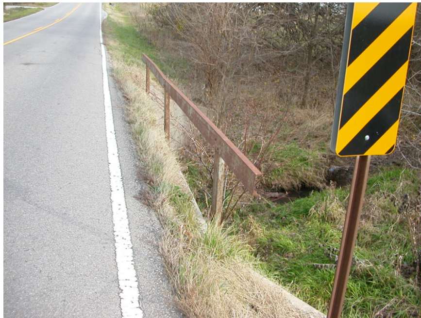
Figure 42.29: Culvert with Zero Offset (Bowers, 2019)
