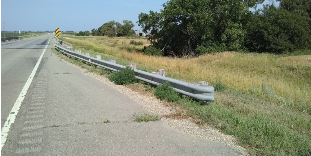
Figure 51.38: Bridge-approach guardrails to Bridge End (Bowers, 2019)
