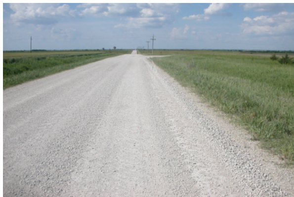
Figure 36.23: Rural Three-or Four-Wheel-Track Gravel or Paved Road (Bowers, 2019)
