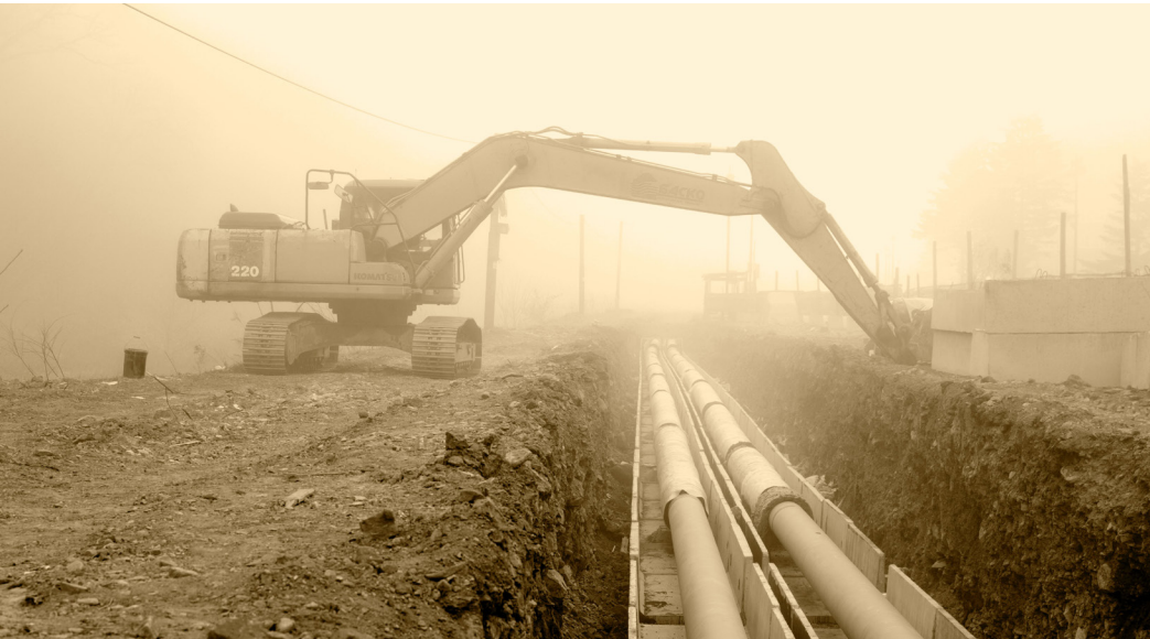
FIGURE 2.01 EXCAVATOR INSTALLING PORTIONS OF PIPELINE (PENTIN 2019).
