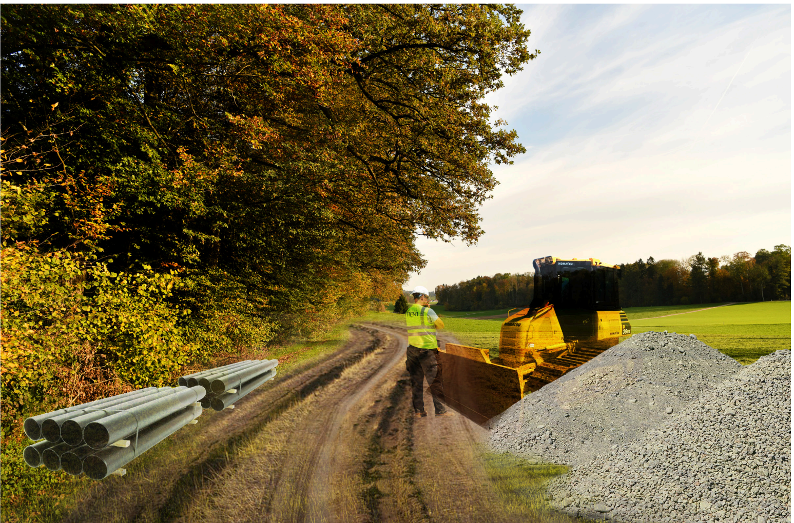
FIGURE 6.13 WIDENED PORTIONS OF THE SULPHUR RIVER CROSSING SEGMENT OF MARKETLINK PIPELINE WERE USED AS CONSTRUCTION STORAGE AREAS, LEADING TO INCREASED SOIL COMPACTION AND EROSION (BAKER 2020)
