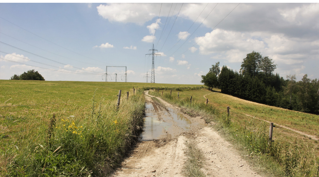
FIGURE 2.03 ACCESS ROAD FOR HIGH-VOLTAGE TRANSMISSION LINE MAINTENANCE AND OPERATIONS (HOSOVA 2019).
