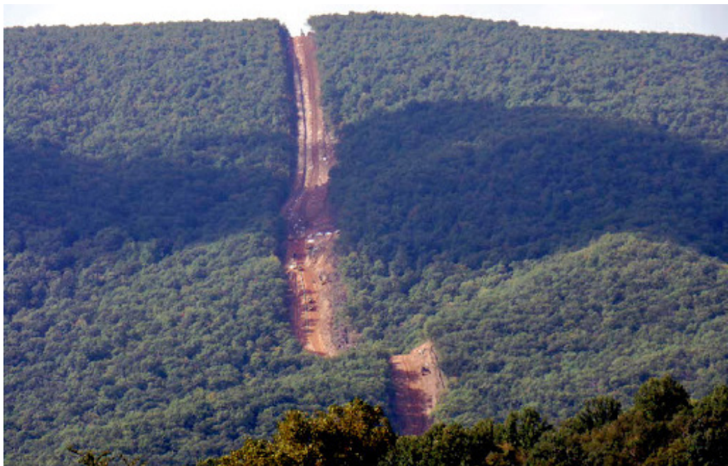
FIGURE 2.00 EXAMPLE OF A PIPELINE RIGHT-OF-WAY CORRIDOR THROUGH THE APPALACHIAN MOUNTAINS (WEBB 2020).
