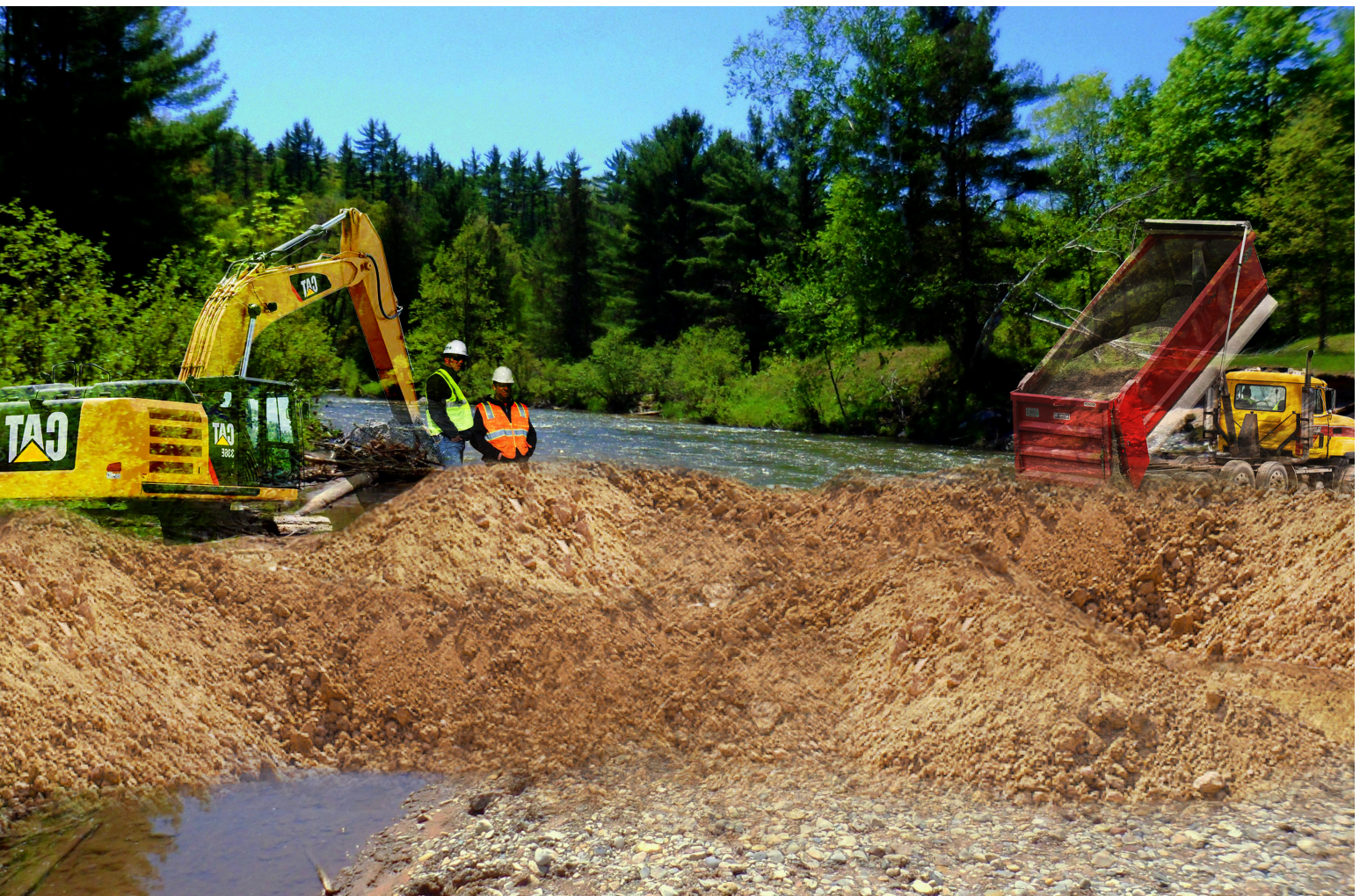
FIGURE 6.18 THIS SEGMENT OF PIPELINE WAS NOT INSTALLED PERPENDICULAR TO THE SULPHUR RIVER STREAM CHANNEL, CAUSING THE STREAM CHANNEL TO DEEPEN AND WIDEN DUE TO ACCELERATED STREAMBANK EROSION (BAKER 2020)
