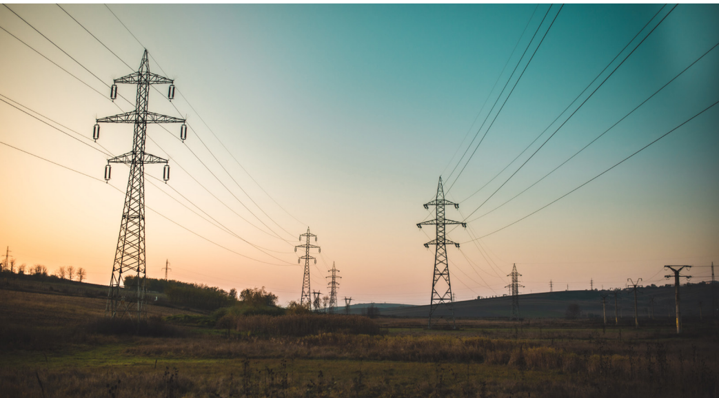
FIGURE 2.02 HIGH-VOLTAGE ELECTRIC TRANSMISSION LINES (BOICU 2019).
