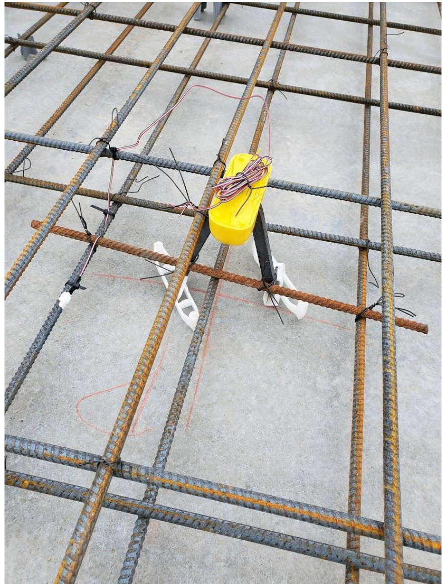
Figure 2-1: Inserts Tied to Rebar
