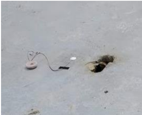
Figure 3-15: Installed Surface Strain Gauge
