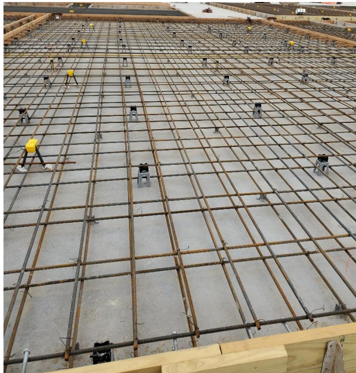
Figure 1-1: Lifting hardware prior to concrete pour
