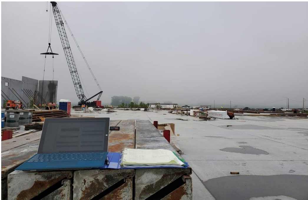
Figure 3-18: Base Station & Laptop Set-Up on Site
