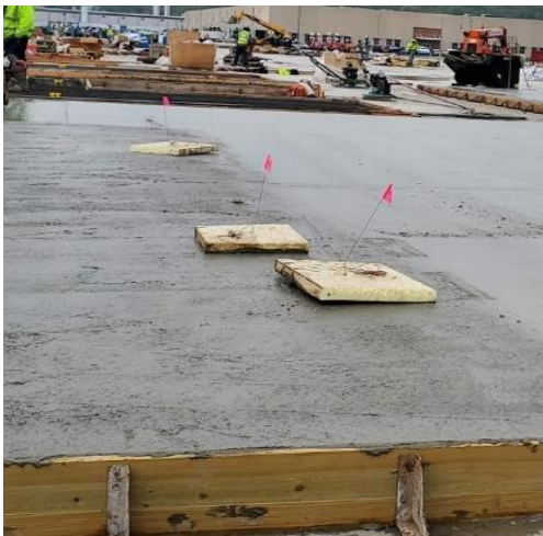
Figure 3-10: Wires Protected in Foam
