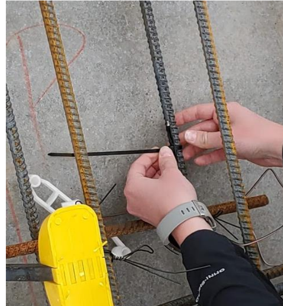
Figure 3-9: Strain Gauge After Being Adhered
