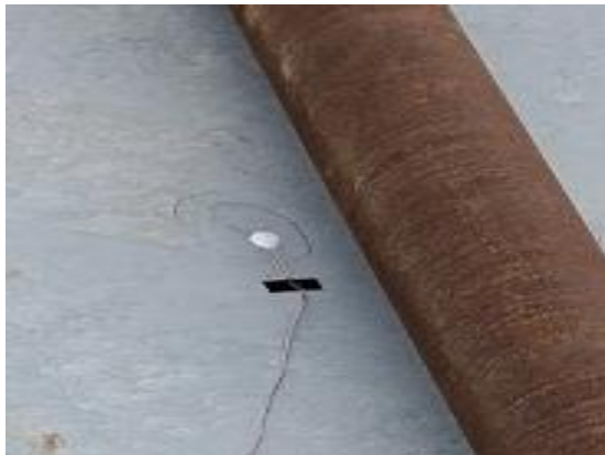
Figure 3-16: Installed Surface Strain Gauge
