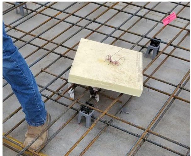
Figure 3-11: Rebar Wiring Protection
