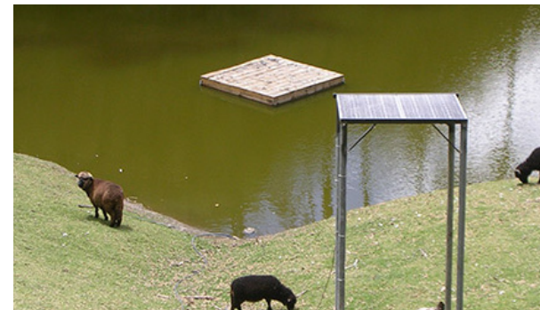
Fig. 4-21. Black Sheep Inn's solar powered pump installed. www.blacksheepinn.com
