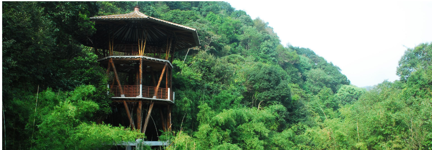
Fig. 4-30. Observation tower designed to expose guests to the environment and weather qualities. Courtesy of EDSA
