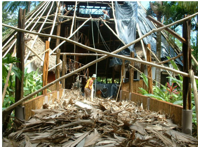
Fig. 4-25. Construction method of thatched roof. www.laparios.com
