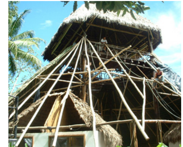
Fig. 3-15. Thatch collected from Lapa Rios site to construct the bungalow roofs. www.laparios.com
