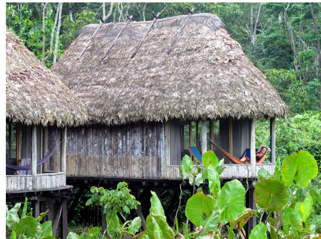
Fig. 4-26. Completed thatched roof construction. www.kapawi.com
