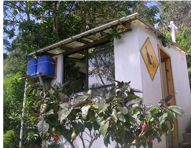
Fig. 3-12. Cisterns collect rainwater from the roof for washing hands. www.blacksheepinn.com
