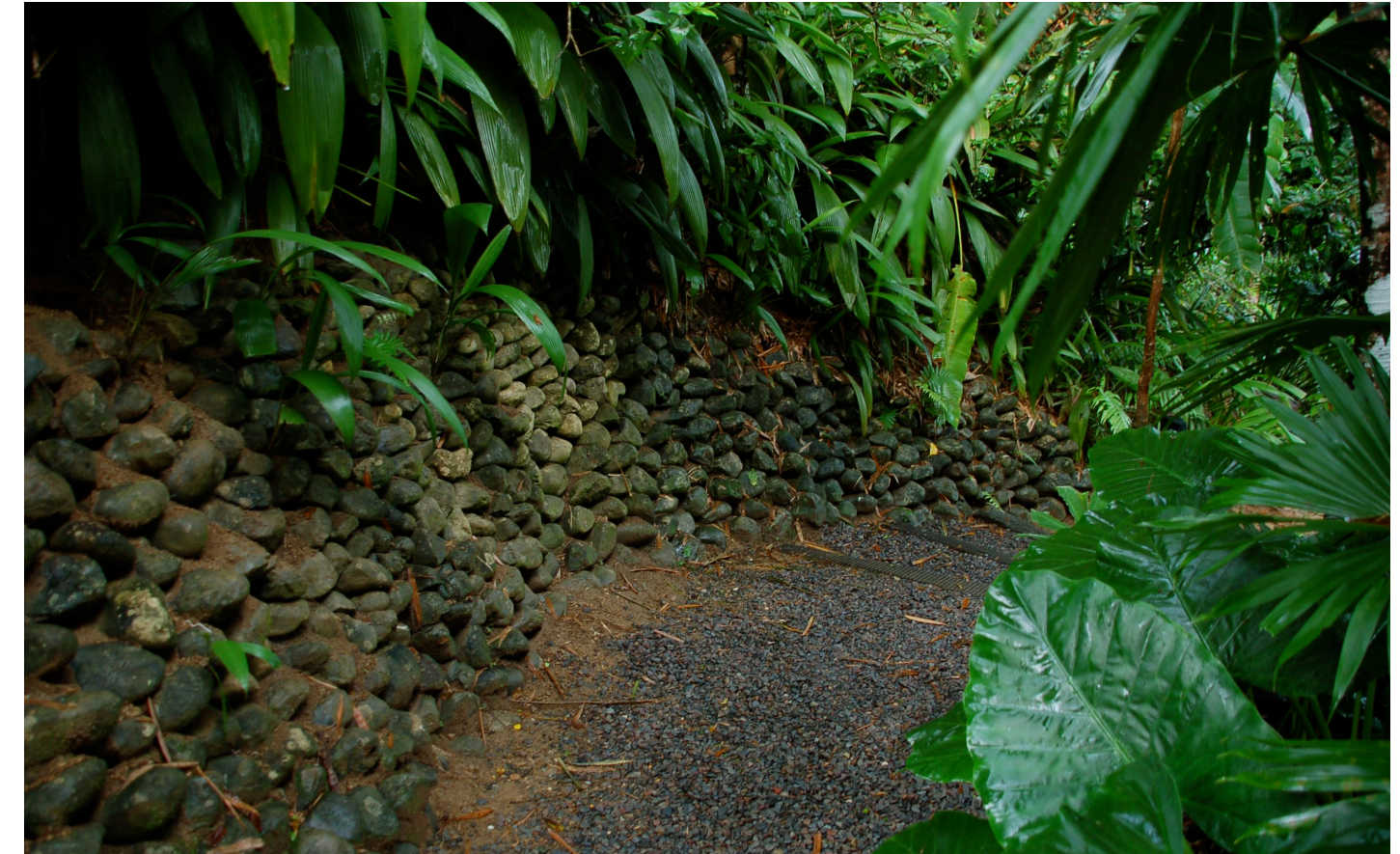
Fig. 3-6. Dry-stacked stone wall on path leading to Lapa Rios suites. Photo courtesy of Mark Dineen.
